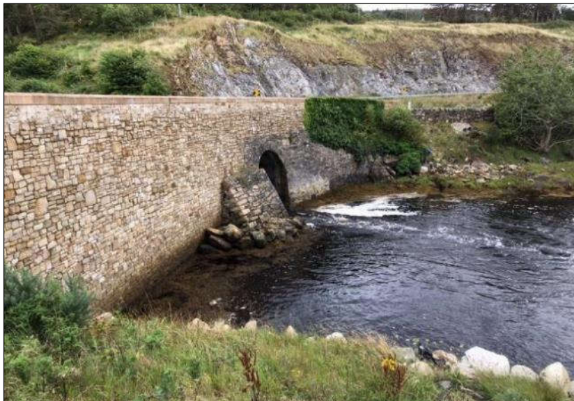
Plate 2-5 Gweebarra Burn Bridge – masonry arch.
