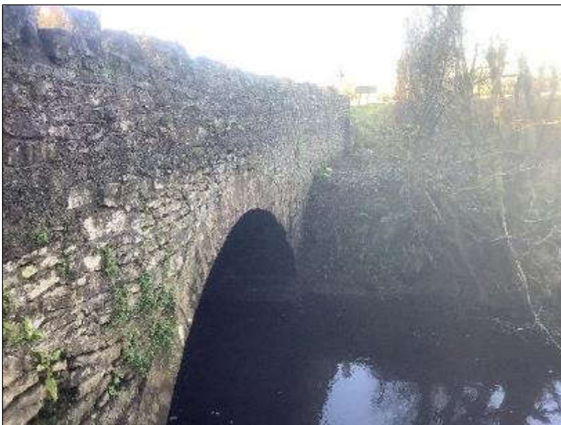
Plate 2-15 Scarden River Bridge.
