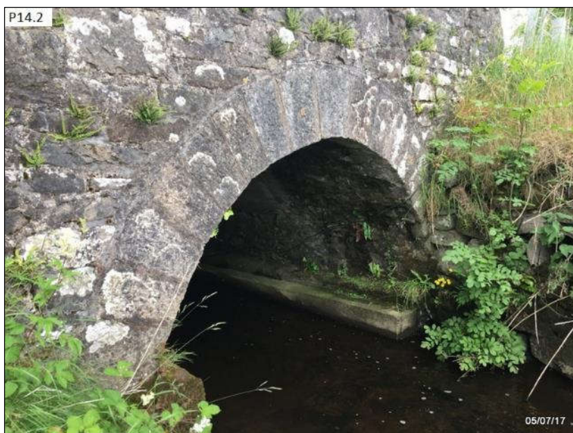
Plate 2-22 Bracklagh Bridge – masonry component.
