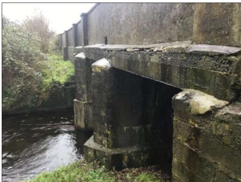
Plate 2-1b Ballachanea Bridge – concrete slab element.
