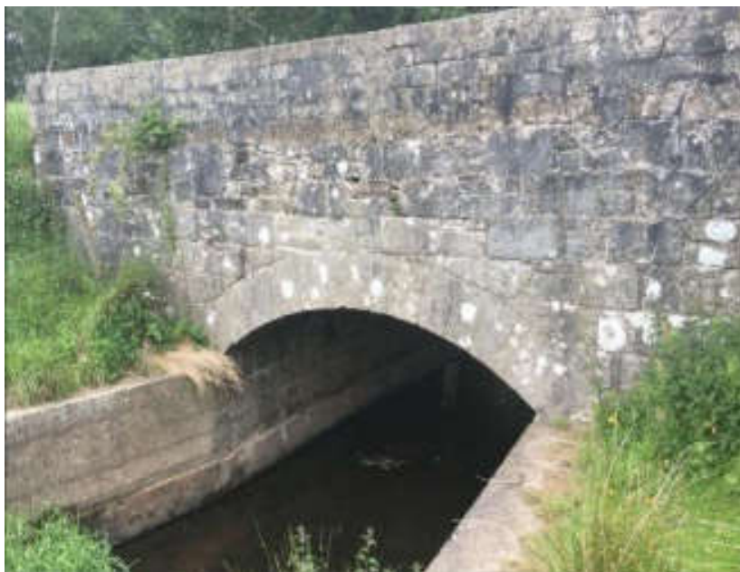
Plate 2-18 Owenmore River Bridge.
