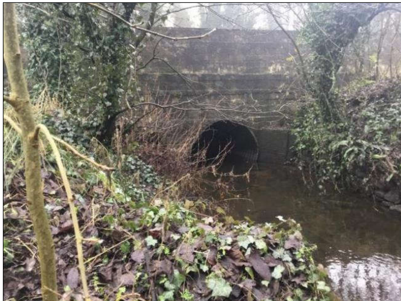
Plate 5-28 Tullybryan Bridge No.2.
