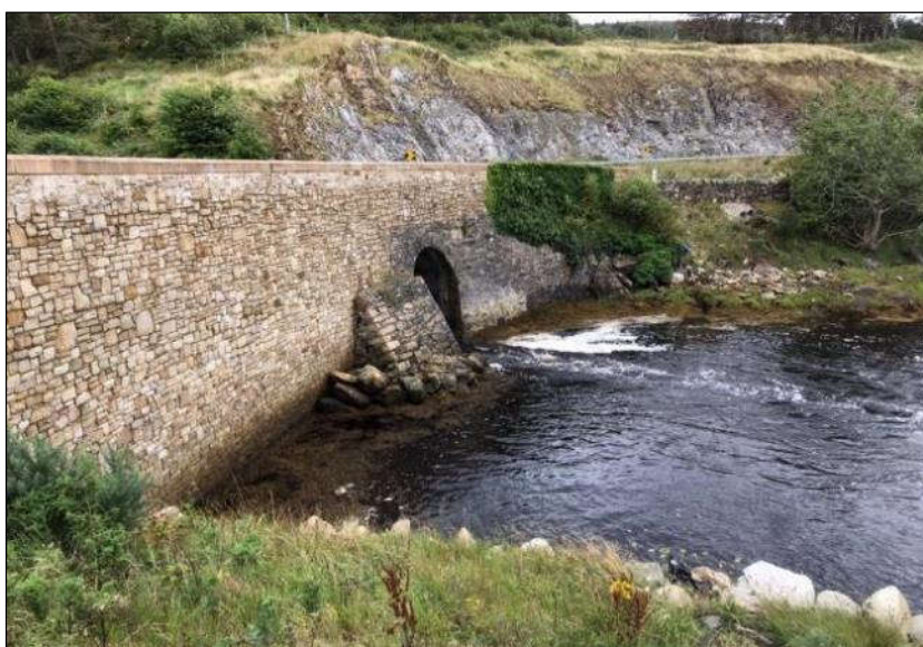
Plate 5-6 Gweebarra Burn Bridge – masonry arch.
