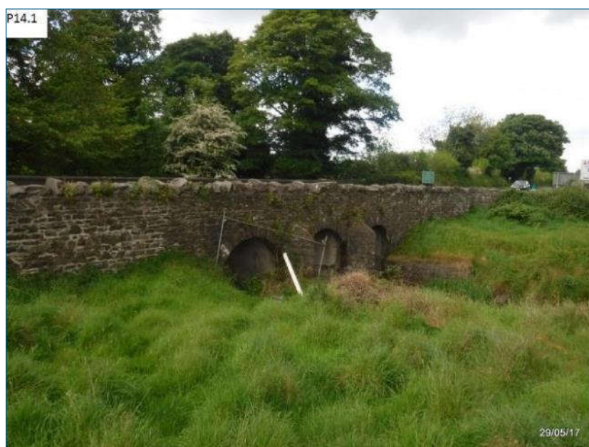
Plate 5-2a Ballachanea Bridge – masonry element.
