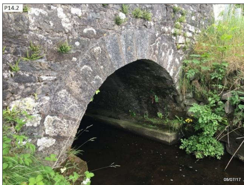
Plate 5-33 Bracklagh Bridge – masonry component.
