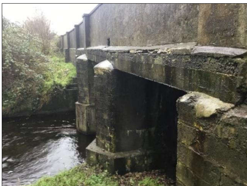
Plate 5-2b Ballachanea Bridge – concrete slab element.
