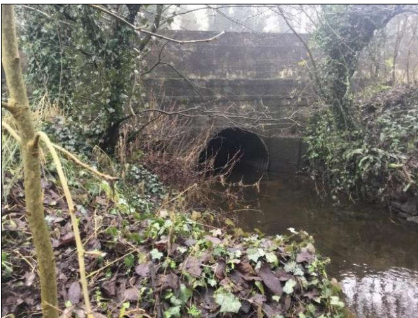
Plate 2-25 Tullybryan Bridge No. 2.
