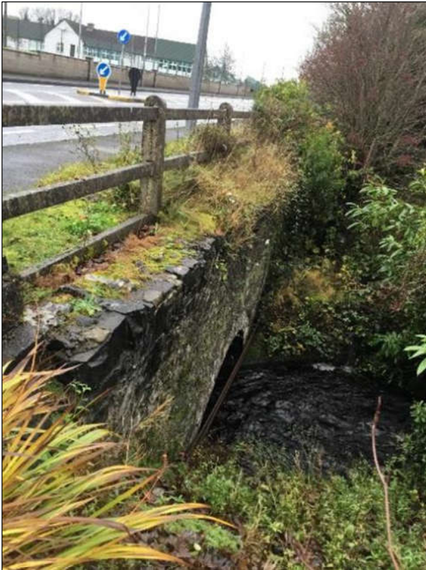
Plate 2-27a Bridge at Yeats Inn, Curry town. Masonry face.
