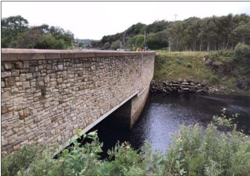
Plate 2-6 Gweebarra Burn Bridge – concrete slab.
