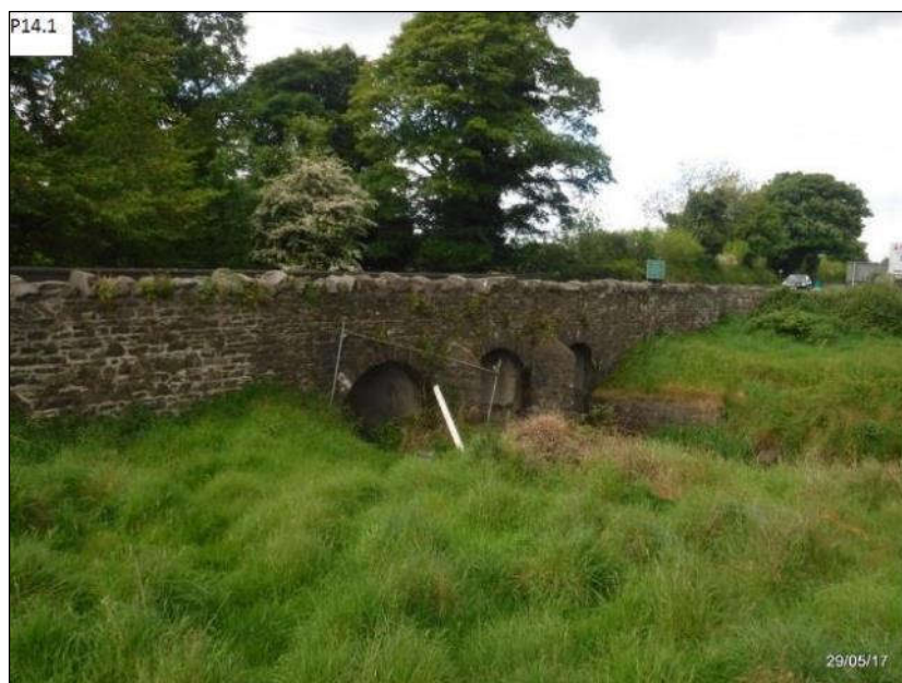
Plate 2-1a Ballachanea Bridge – masonry element.
