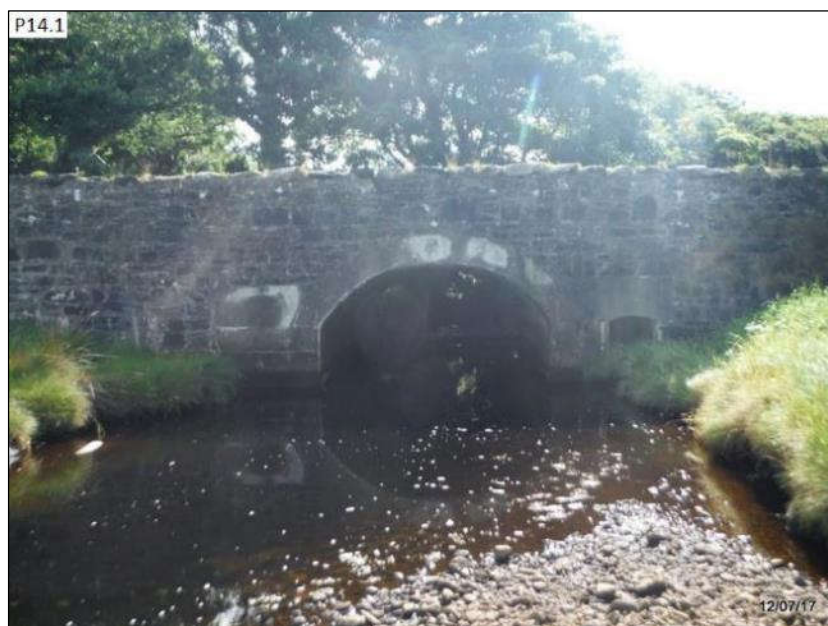
Plate 5-9 Barnaderg Bay Bridge No.2.
