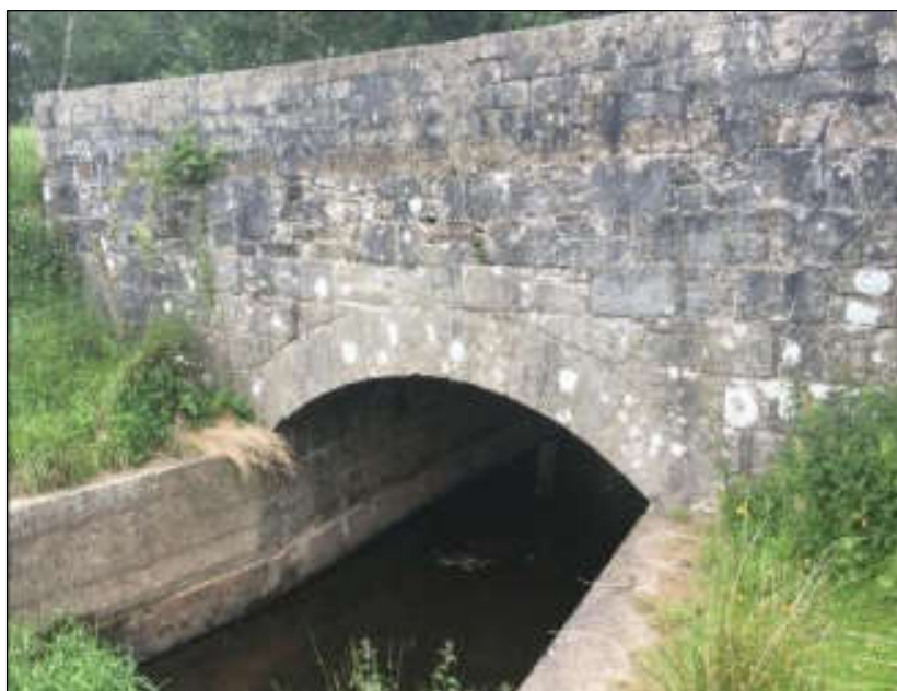
Plate 5-19 Owenmore River Bridge.
