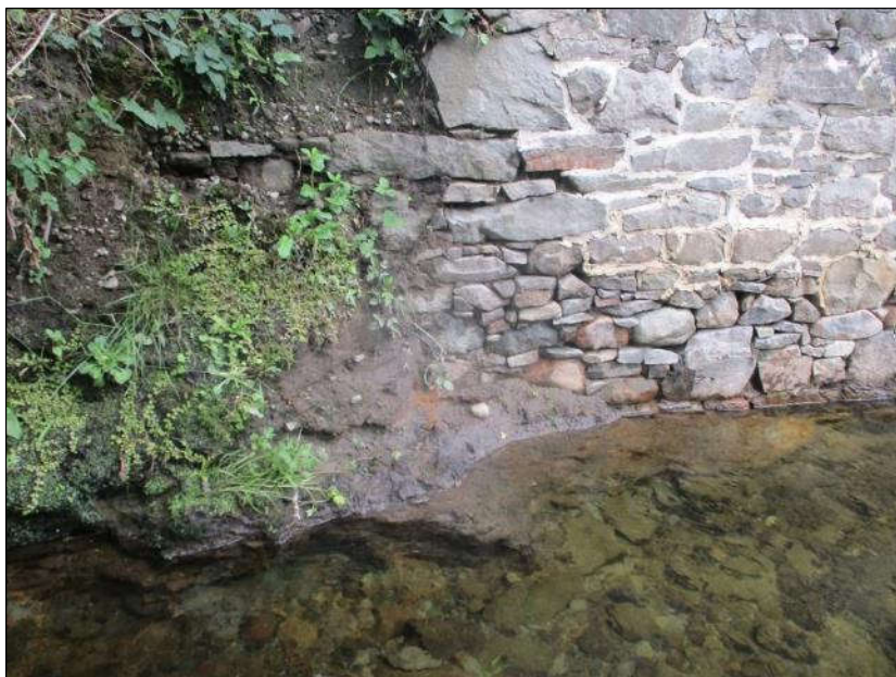
Plate 5-27 Mud to be removed.
