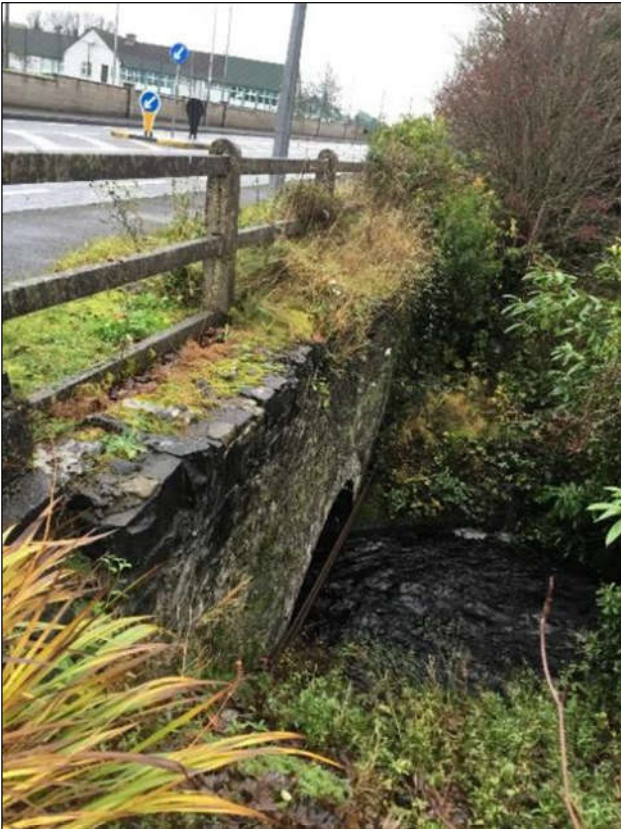
Plate 2-30a Bridge at Yeats Inn, Curry town. Masonry face.
