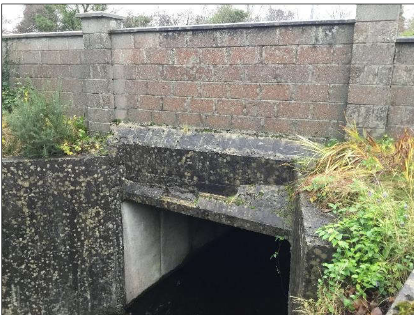
Plate 2-27b Bridge at Yeats Inn, Curry town. Concrete slab face.
