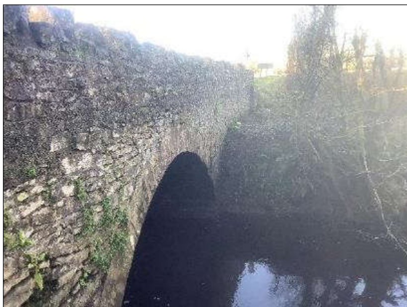
Plate 5-16 Scarden River Bridge.
