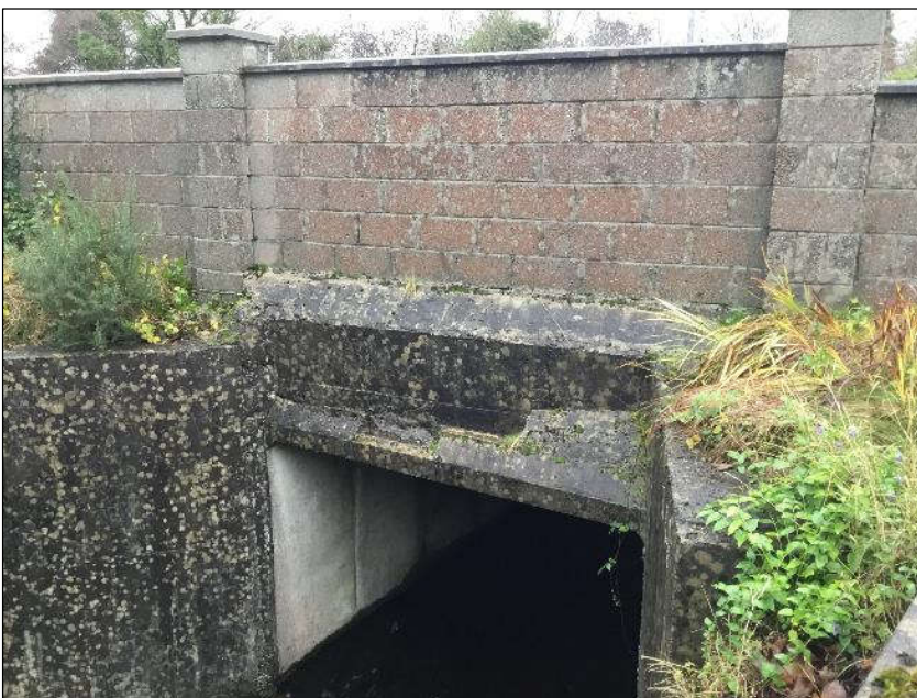
Plate 2-30b Bridge at Yeats Inn, Curry town. Concrete slab face.
