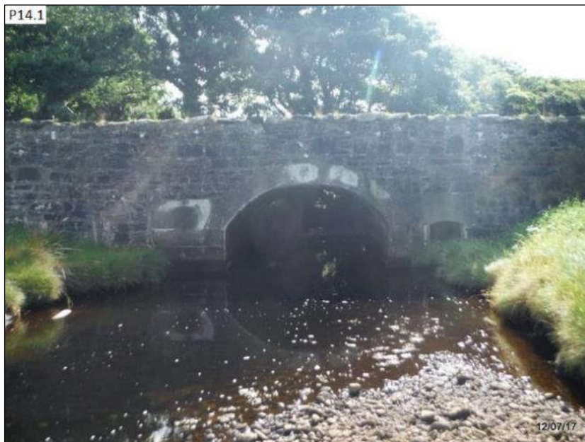
Plate 2-8 Barnaderg Bay Bridge No.2.
