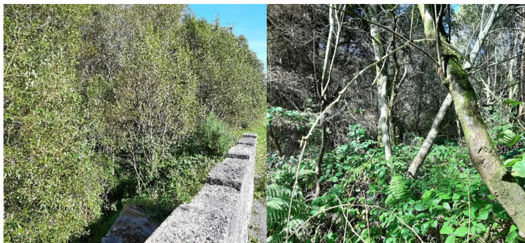
Plate 4.2: Upstream of Coolturk Bridge.
