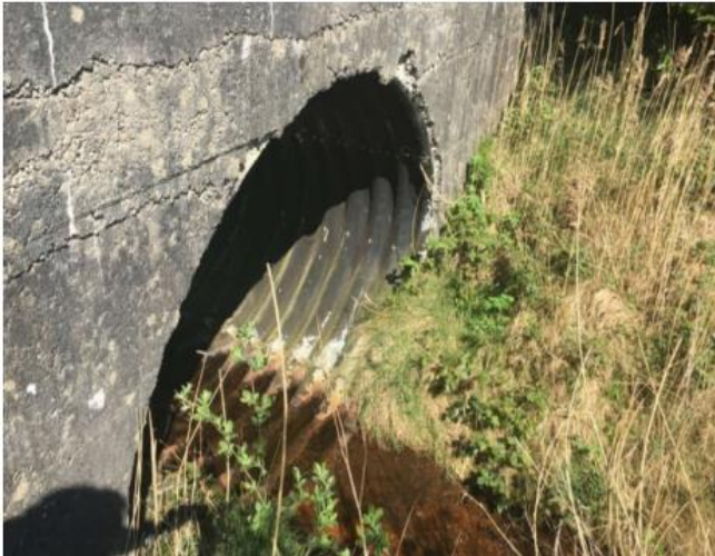
Figure 3-1 – Coolturk culvert at exit
