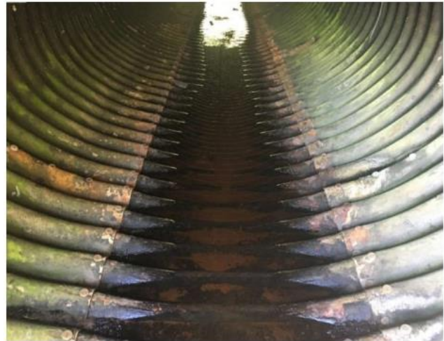
Figure 3-2 – Inside view of the culvert
