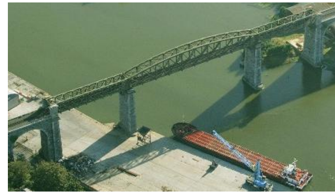
Boyne Structural Assessment
