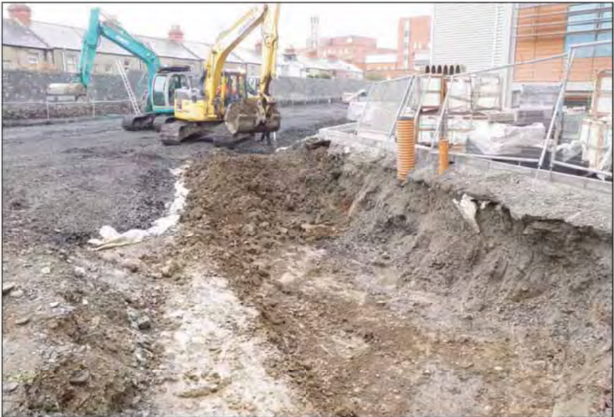
Plate 24. Monitoring of stop-box guide wall excavation along western boundary facing south-east.
