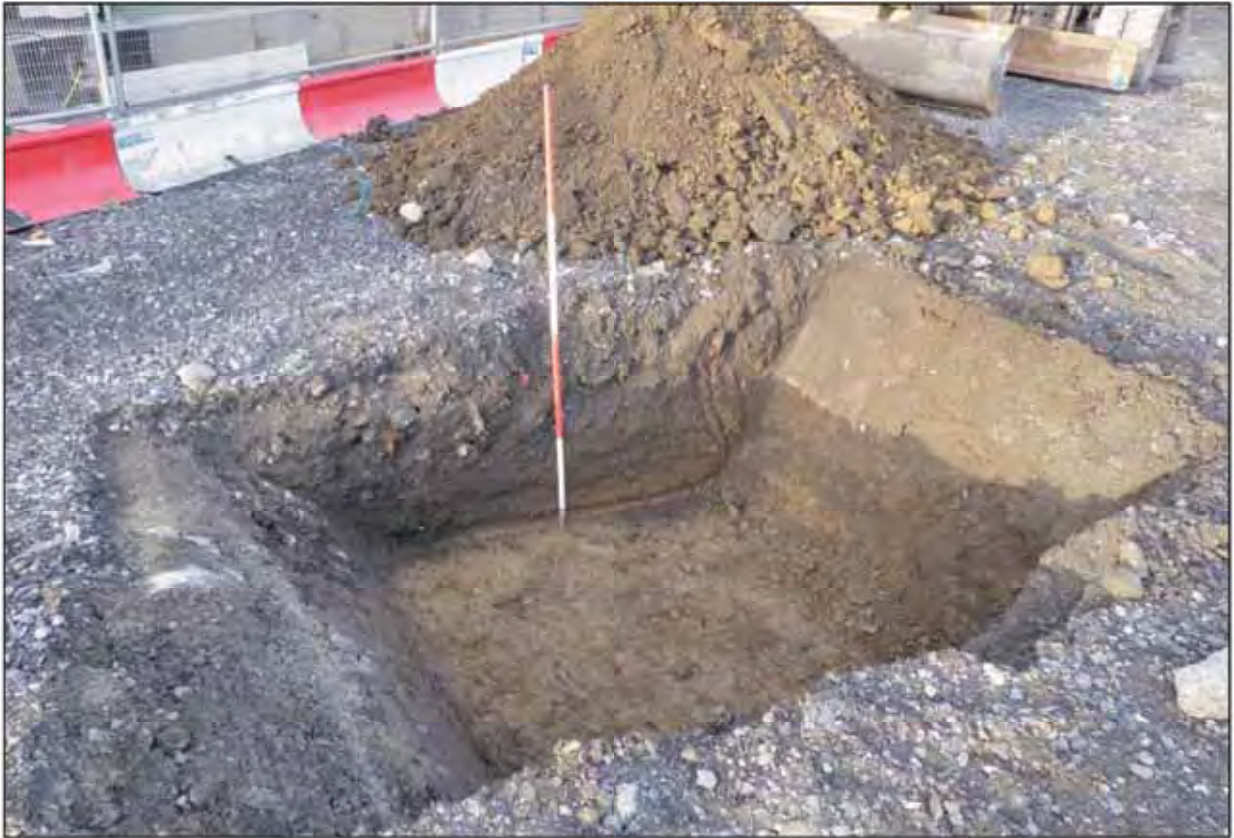
Plate 13. Site Investigation Test Pit 1 facing northwest.
