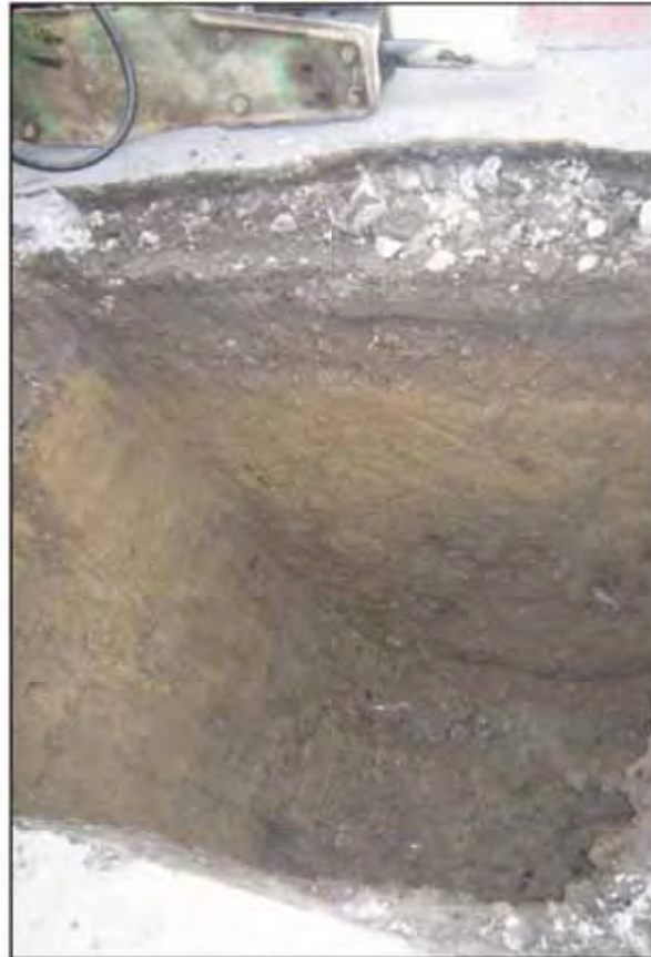
Plate 17. Site Investigation Test Pit 5 facing south.
