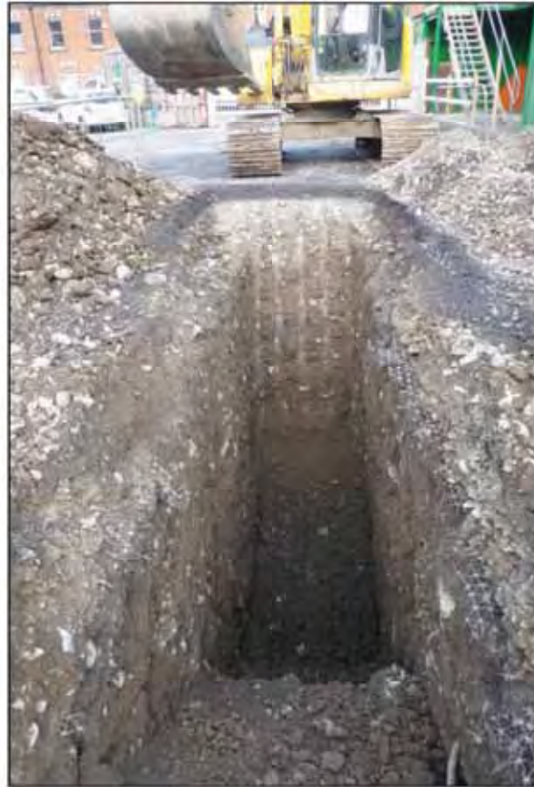
Plate 3. Made ground identified in northern extent of Test Trench 1.
