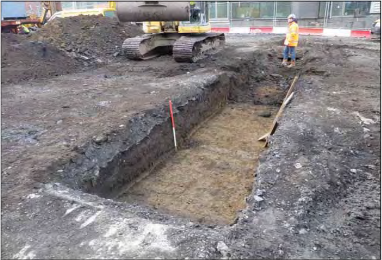
Plate 11. Test Trench 5 facing west.
