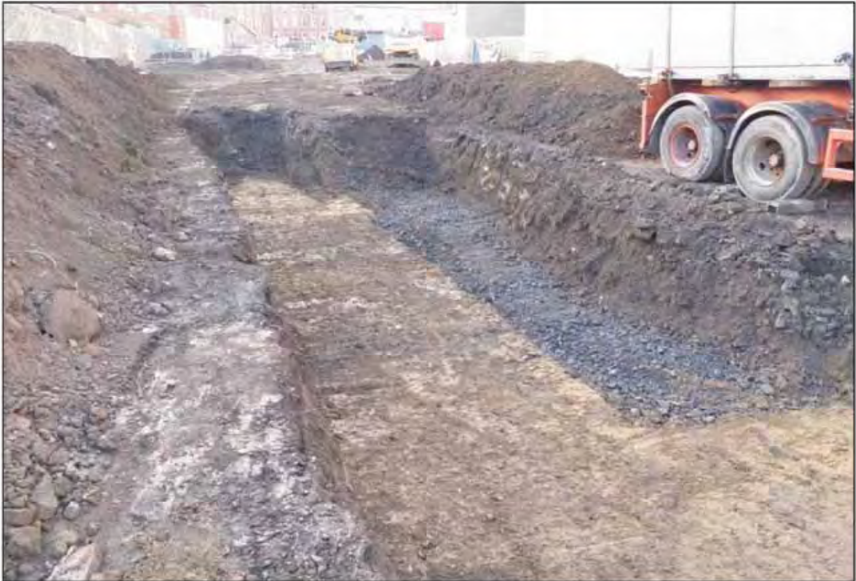
Plate 21. Monitoring of overburden removal through centre of the site facing south.
