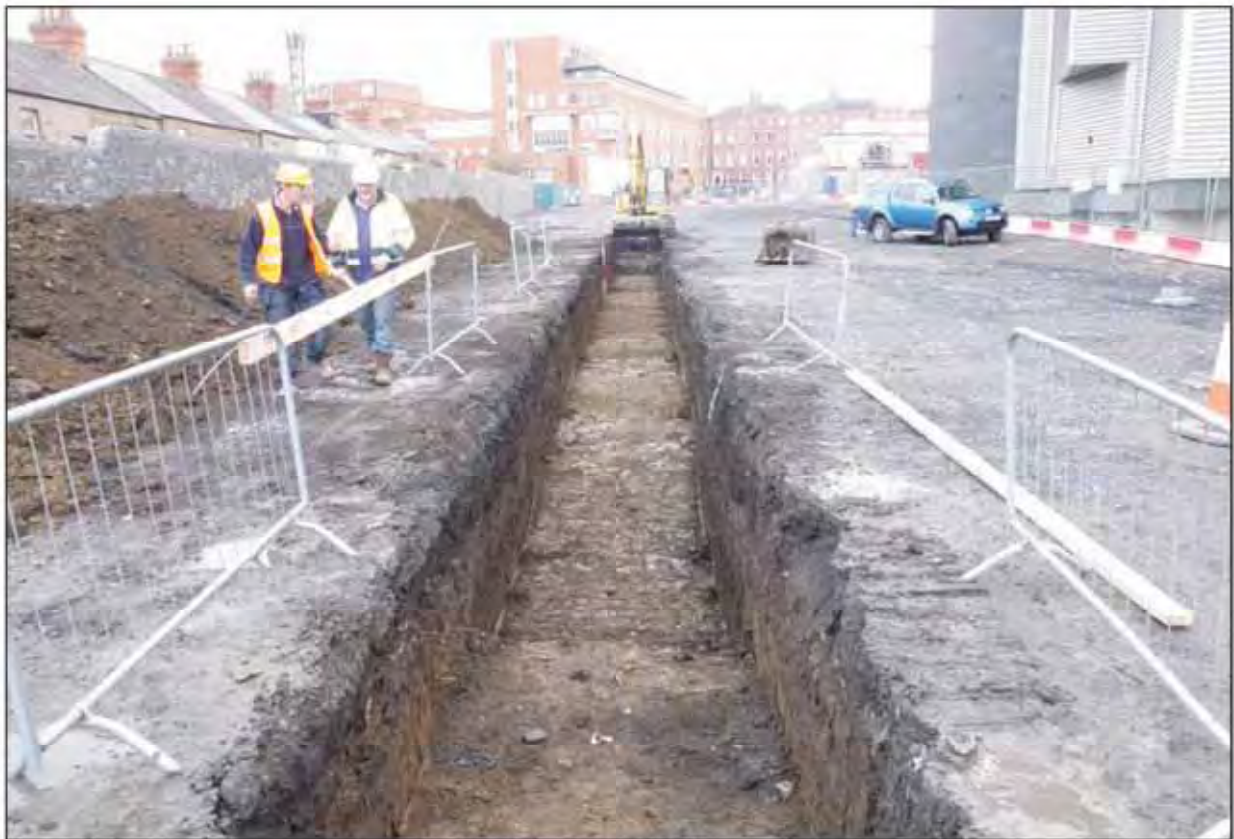
Plate 2. Test -Trench 1 facing south.
