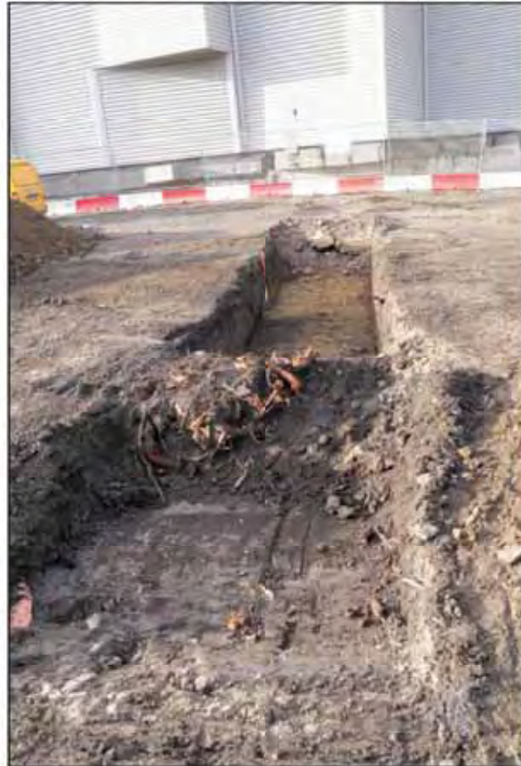
Plate 7. Test Trench 3 facing west, note tree trunk at eastern extent.
