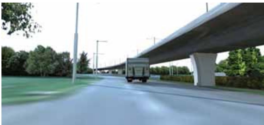
Viaduct at Pinnock Hill Roundabout
