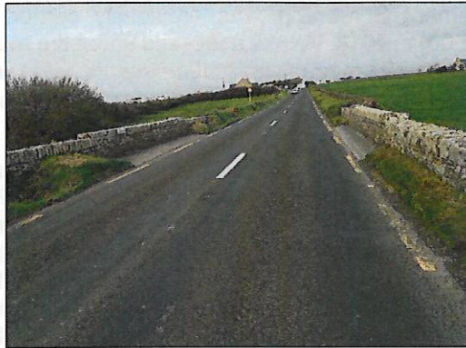
Plate 1. Kilmurry Bridge. View from deck [Source: Atkins R.E.; 26/10/2018].
