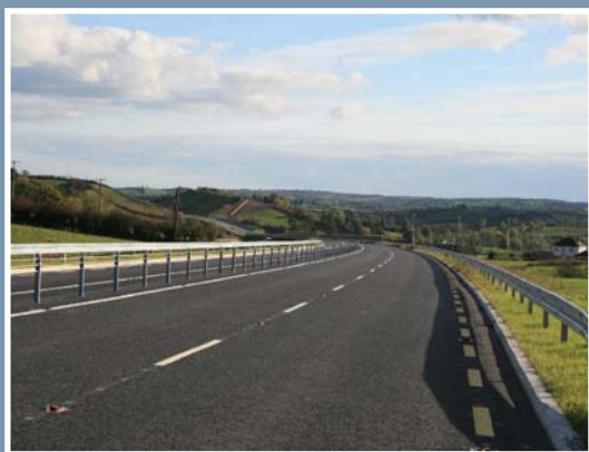
▶ N2 Castleblaney bypass, completed 2007
