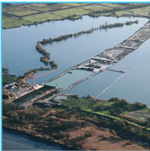
▶ N7 Limerick Tunnel, under construction (PPP scheme)
