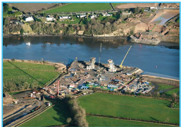
▶ N25 Waterford City Bypass, under construction (PPP scheme)
