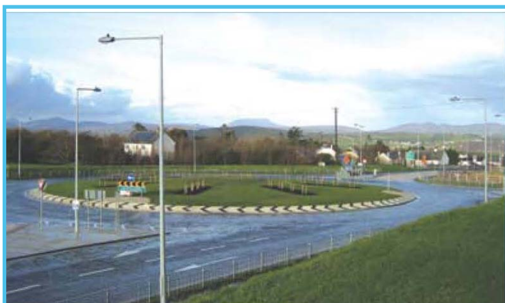
▶ N56 Mountain Top to Illistrin, completed 2007
