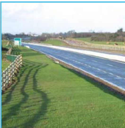
▶ N18 Ennis Bypass, completed 2007
