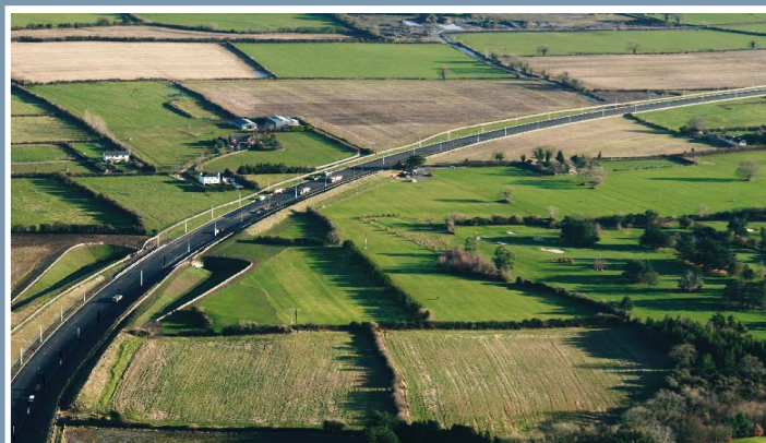
▶ N77 Kilkenny Ring Road Extension, completed 2007
