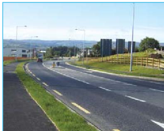
▶ N56 Mountain Top to Illistrin, completed 2007
