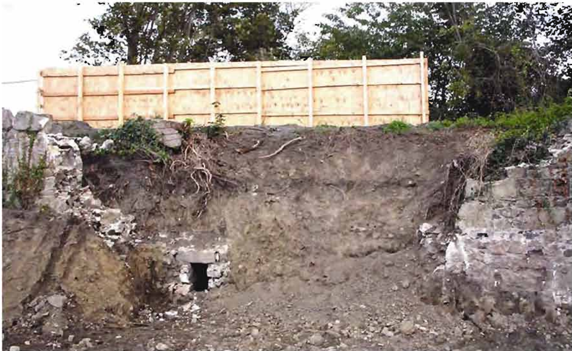
Plate 24: Brenanstown Site 6. Photograph showing stone lined culvert behind embankment wall. Facing north.
