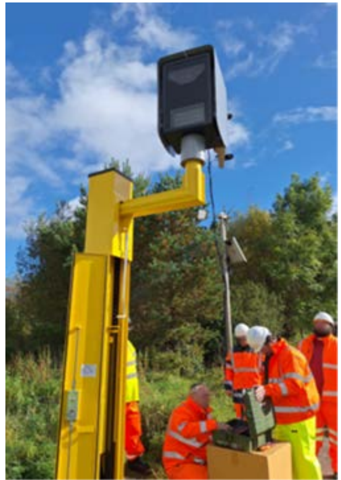
Image: Installation of an N5 average safety camera Co. Mayo September 2024.
