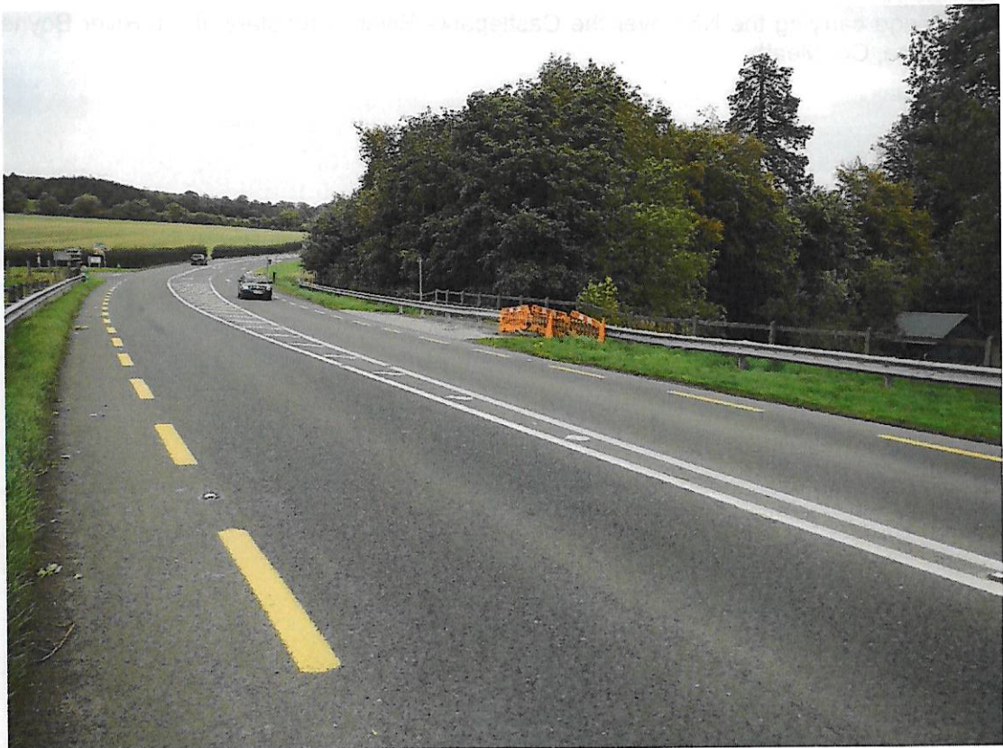
Plate 1. Slane Castle Bridge
