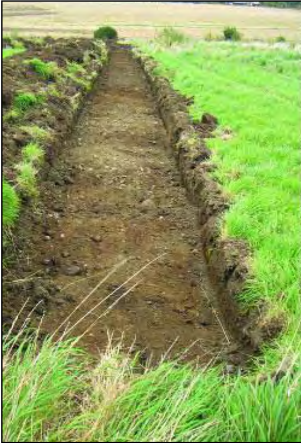
Plate 1 - General photograph of Test Trench 3, Sub-area 22 showing field drain in foreground, looking northeast
