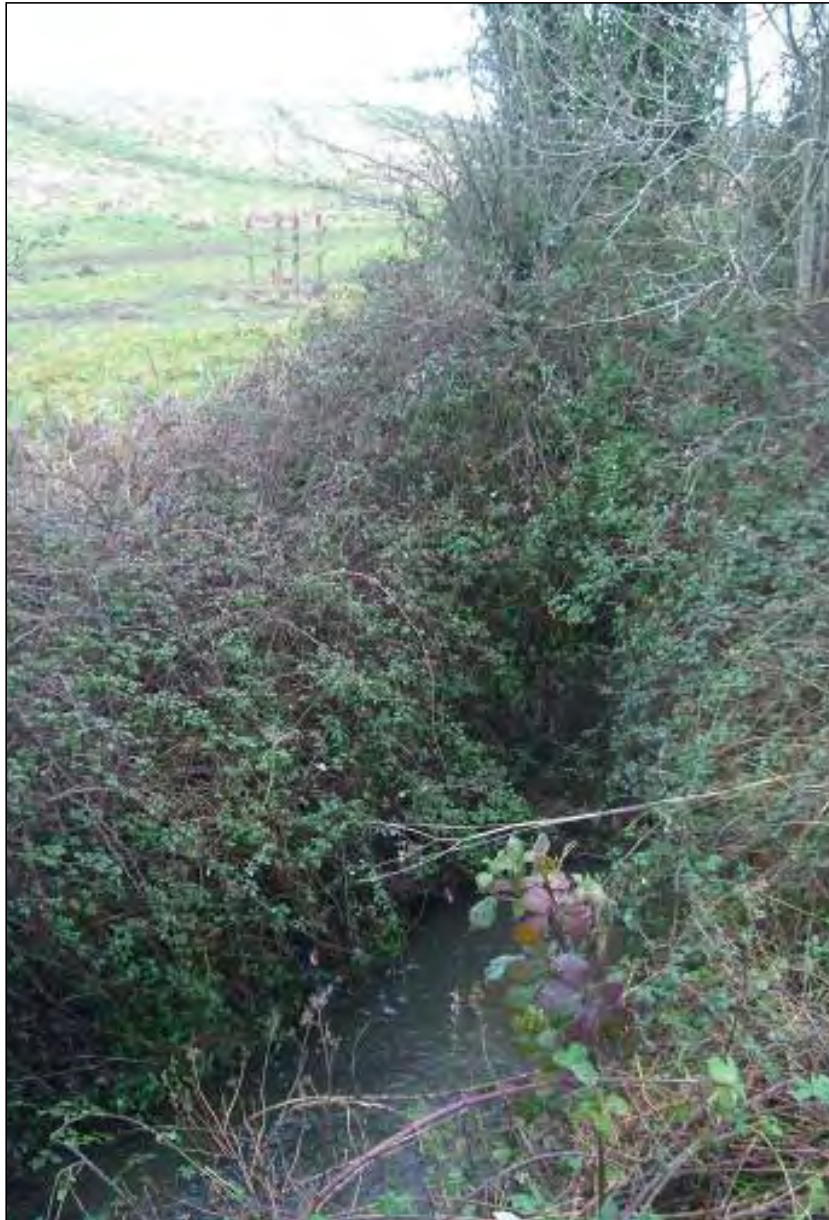
Plate 12 - Photograph of fast flowing stream at base of townland boundary (HC#417) ditch (Sub-area 23) looking northeast.
