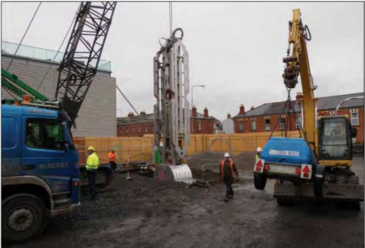
Plate 28. Hydromill excavating Mater D-Wall test panel facing north-west.
