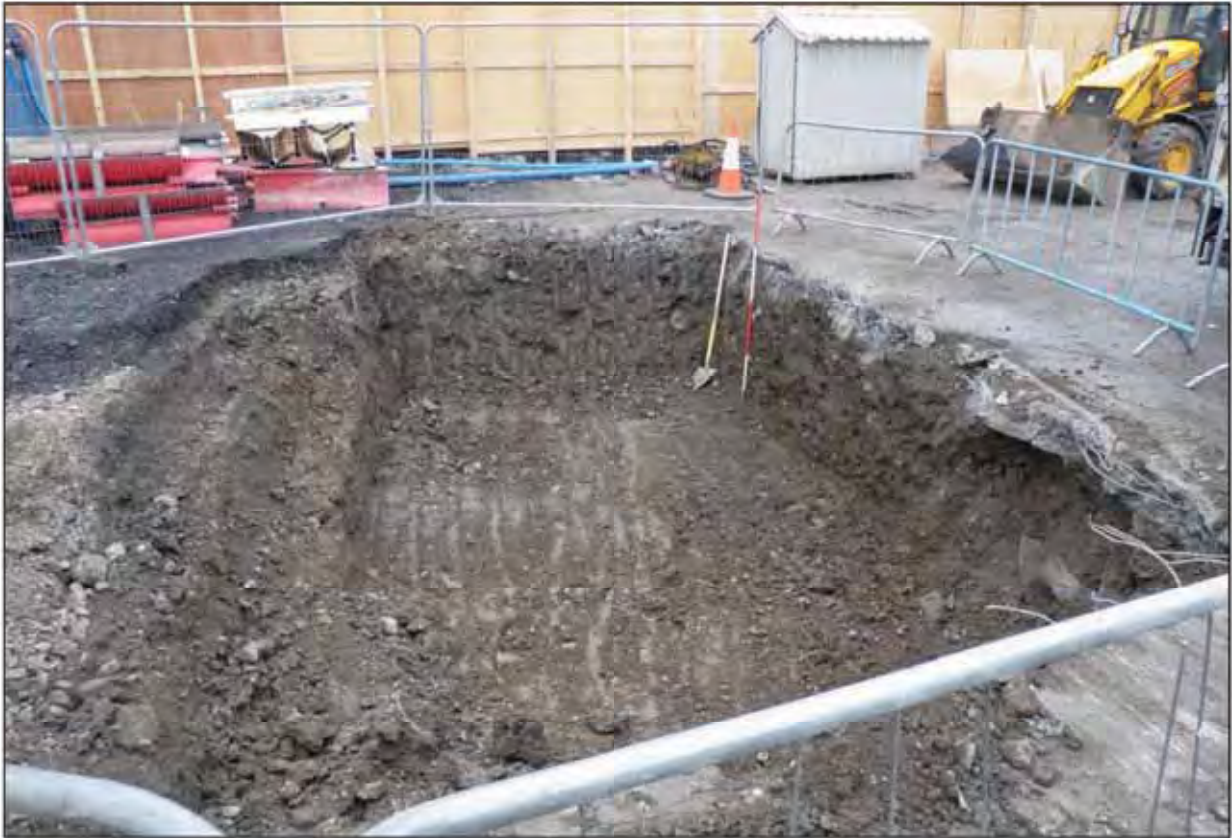
Plate 27. Mater D-wall test panel excavation facing west.
