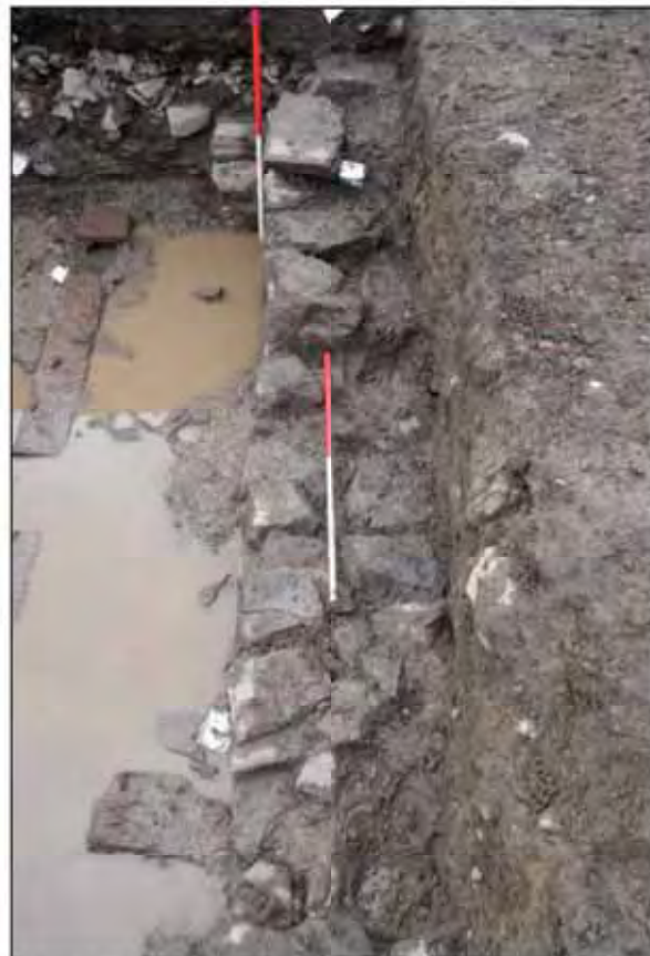
Plate 30. Northern wall (026) of culvert (005) facing west.
