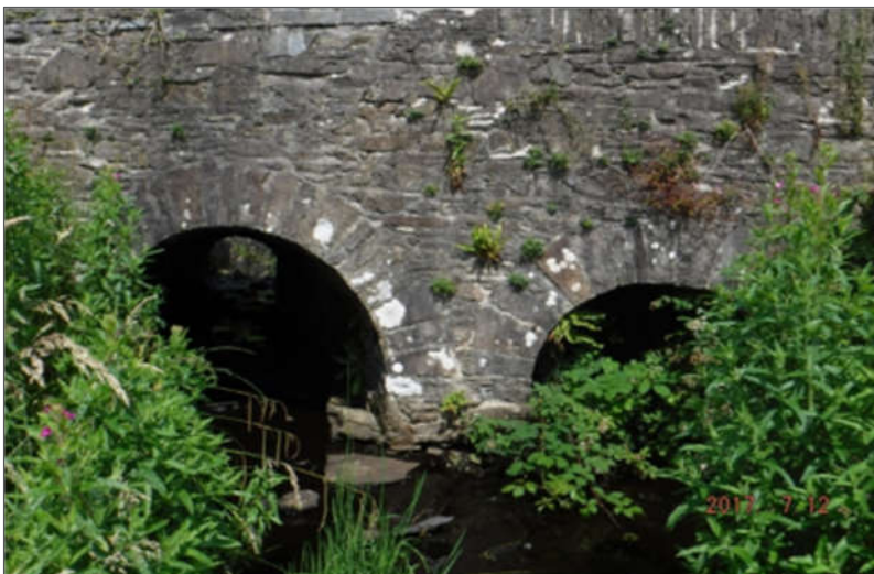
Plate 2-2 Liscasey Bridge West.
