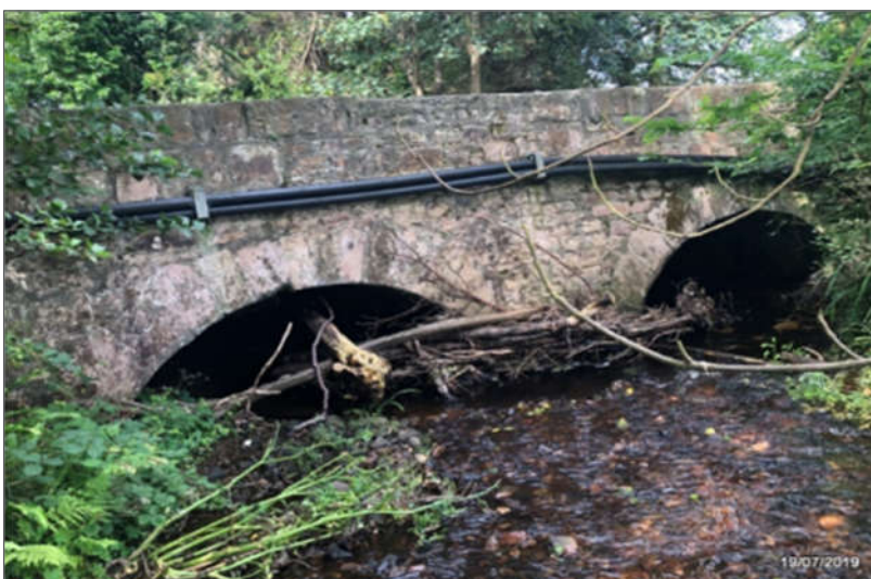
Plate 5-13 Kilfeighny North Bridge.
