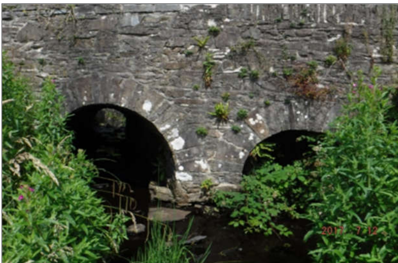
Plate 5-2 Liscasey Bridge West.
