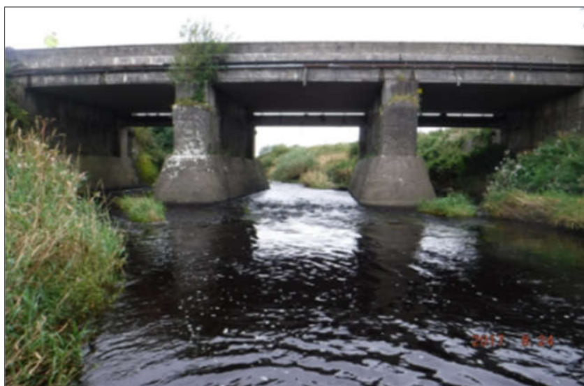
Plate 5-11 River Galey Bridge.
