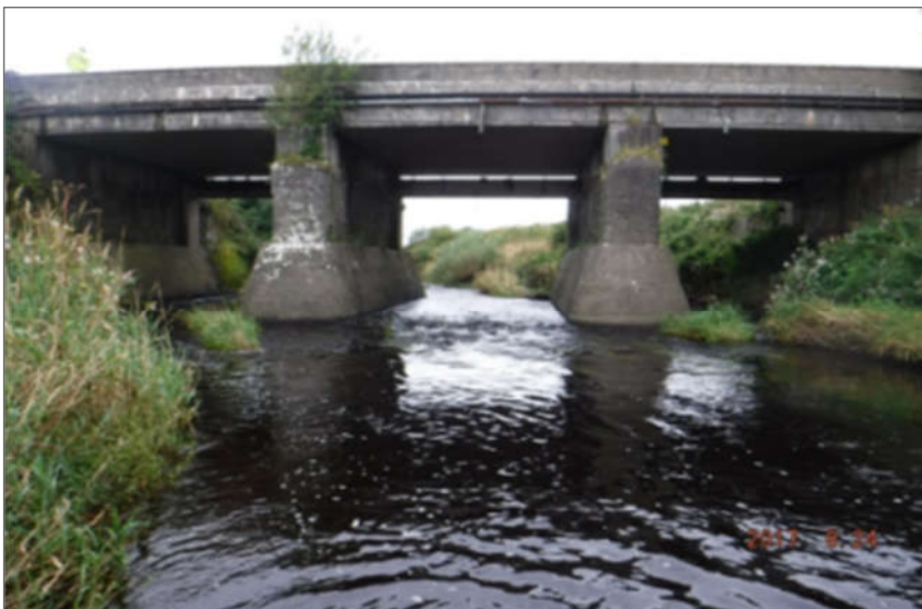
Plate 2-11 River Galey Bridge.
