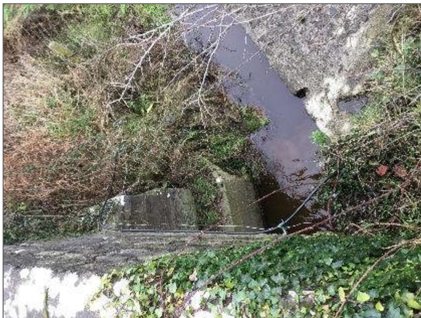
Plate 2-12 Galey Bridge Culvert.
