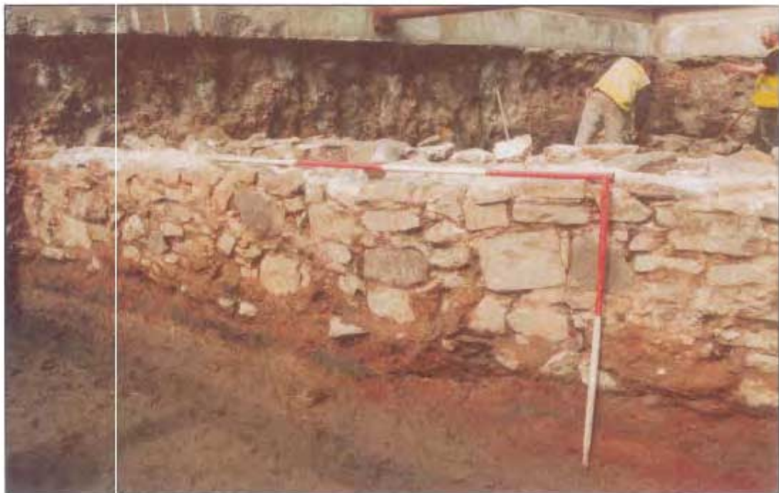
Plate 2 Feature 1, quay wall, facing northwest
