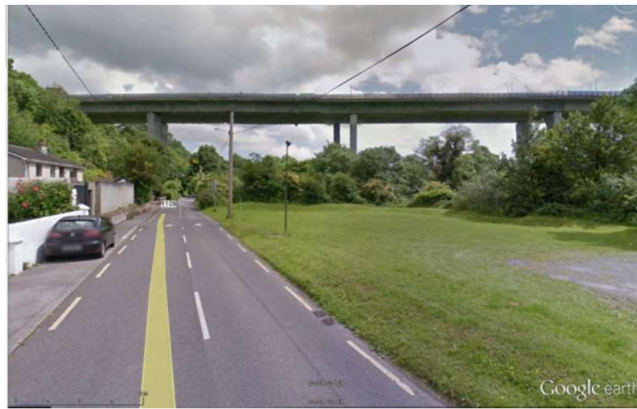
Figure 7 - M50 West Link Bridge across the Liffey Valley at Strawberry Beds
