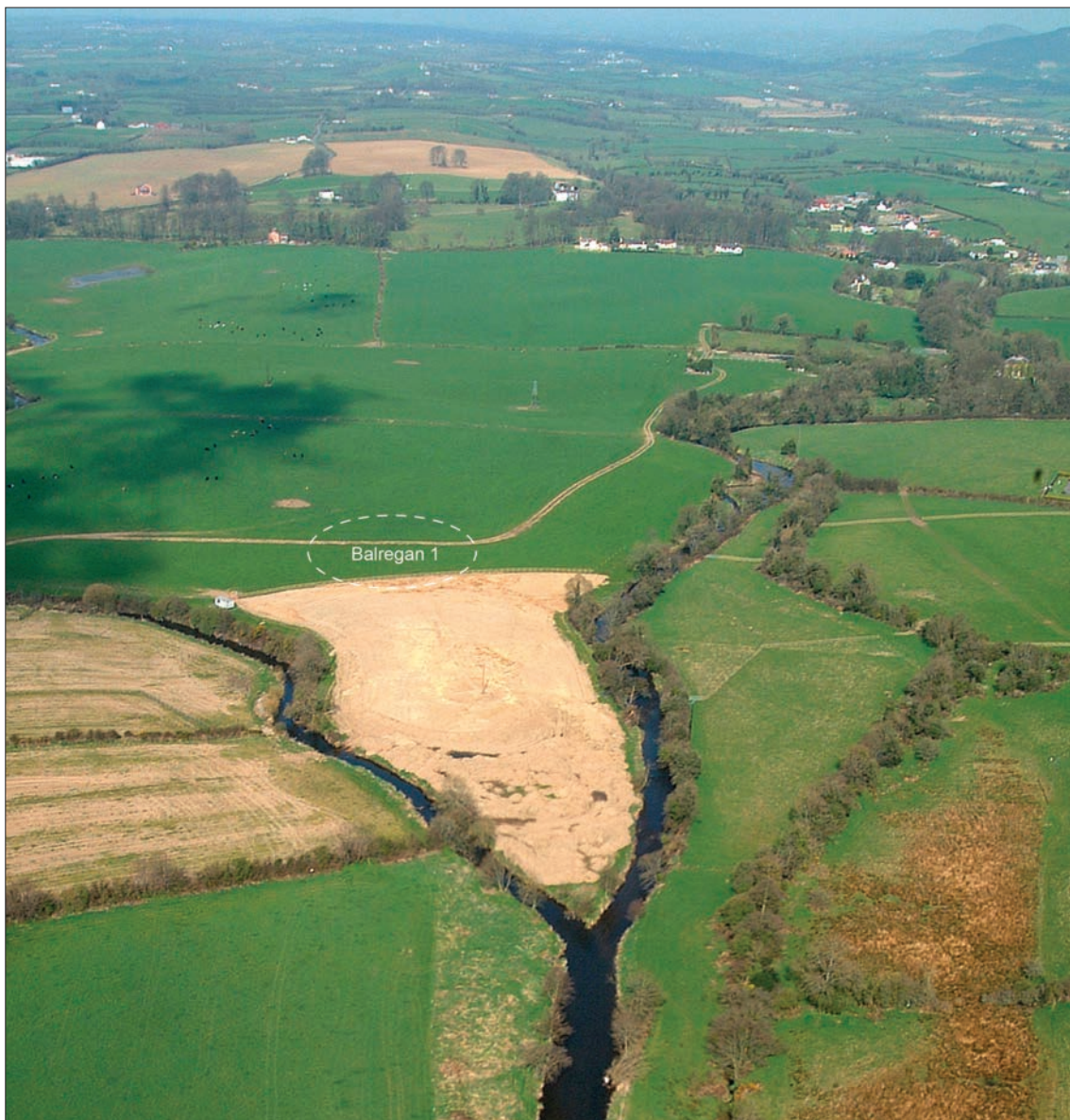
Illus. 8—Aerial view of the Balregan enclosure at the confluence of the Castletown and Kilcurry rivers (Studio Lab).
