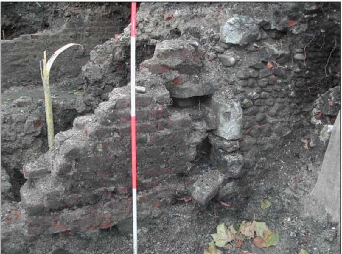
Plate 2 Cobble wall (right) at its junction with the brick latrine wall. Note protruding intermediary masonry blocks
