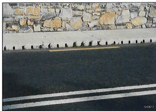
Plate 4. Kerb drainage at Rossow Bridge.
