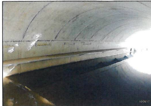
Plate 4. Arch of Rossow Bridge showing no outfall through bridge deck.
