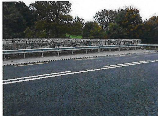
Plate 1. Rossow Bridge. View from deck.
