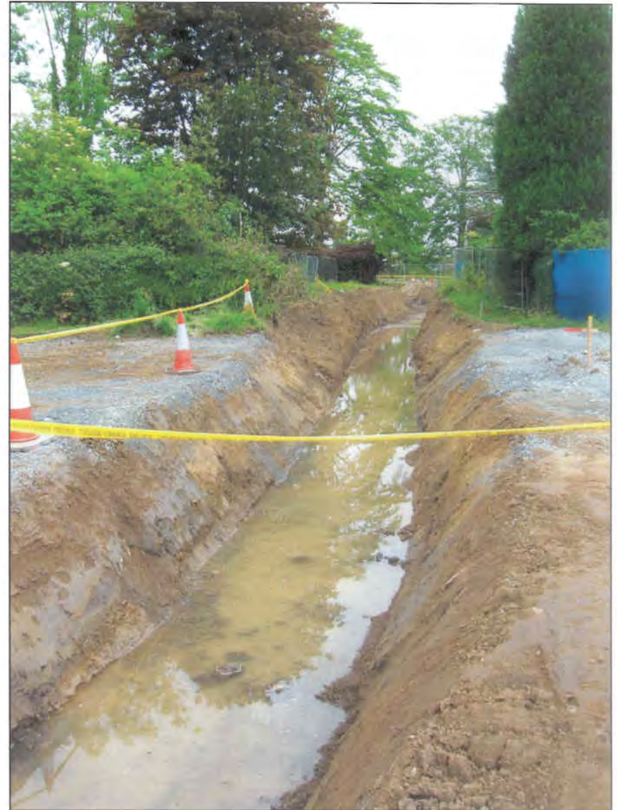
Plate 4 View E of diverted culvert
