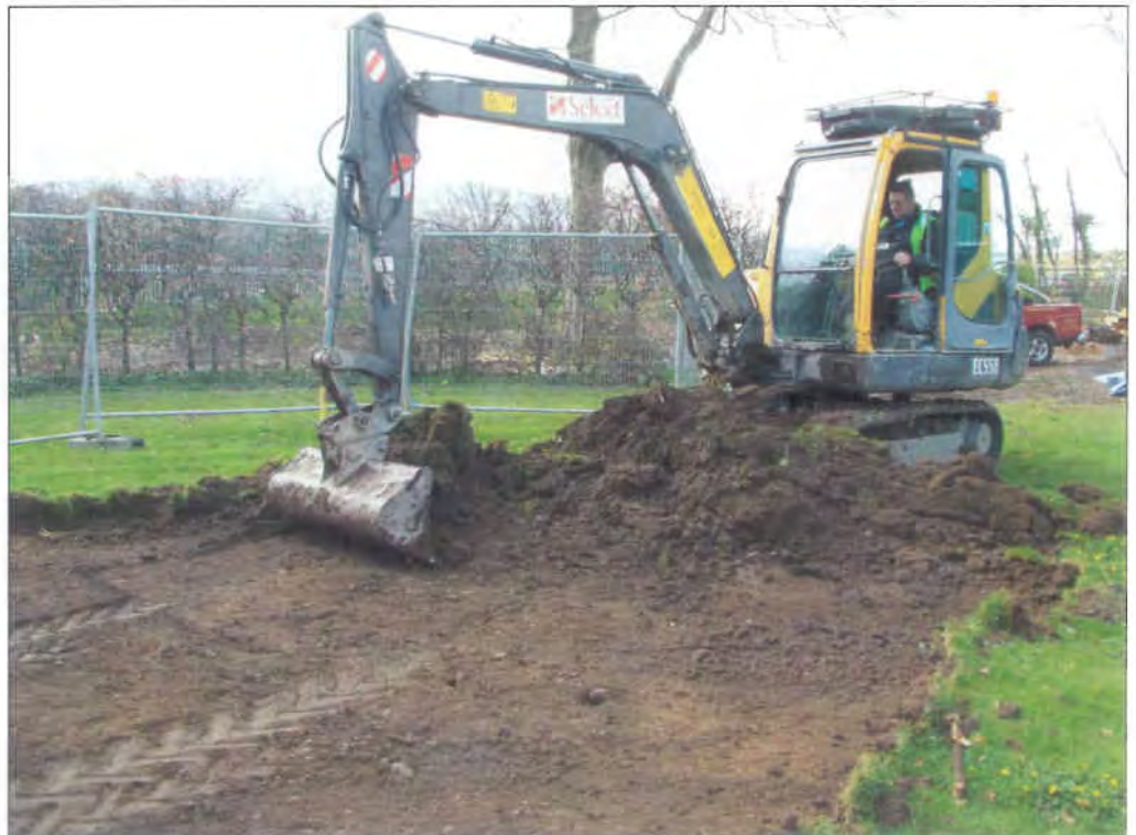
Plate 2 Removal of topsoil with mechanical digger
