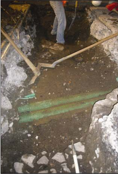
Plate 5 - Mid-ex of disturbed deposit (012), ST720, D'Olier St., west-facing.
