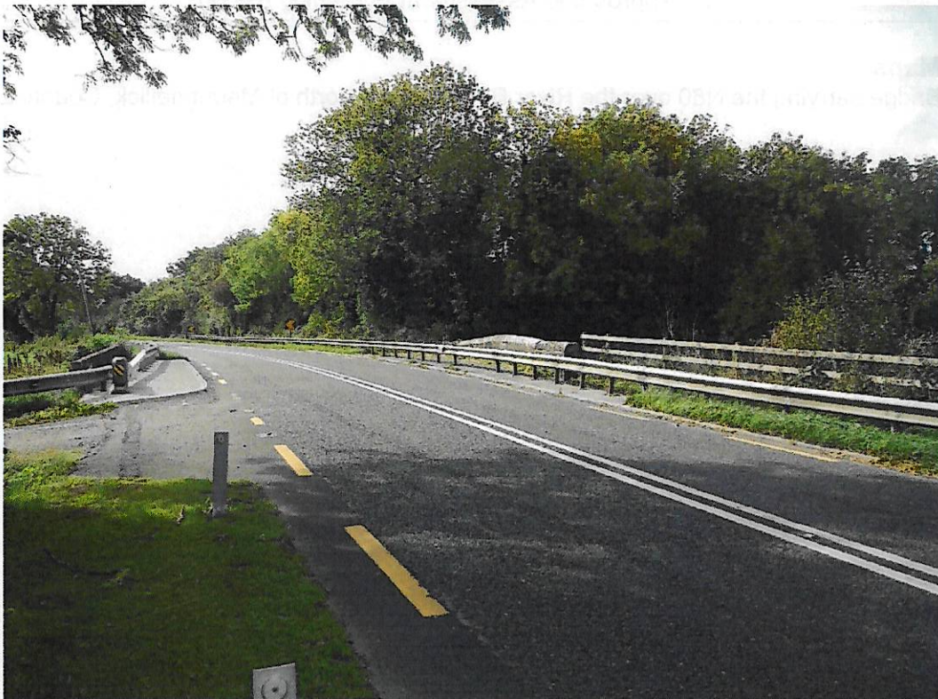
Plate 1. Two Mile Bridge
