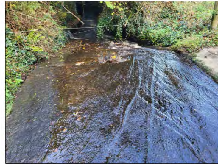
3. NORTHERN APRON LOOKING NORTH
