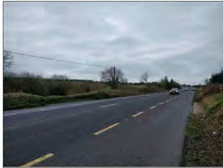
1. EAST APPROACH TO STRUCTURE
