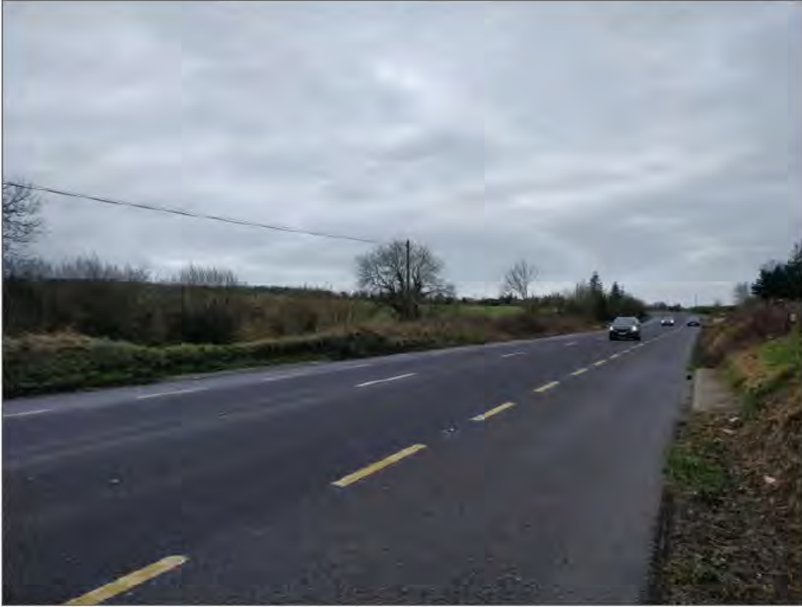
Plate 1-1 Bridge approach from east.
