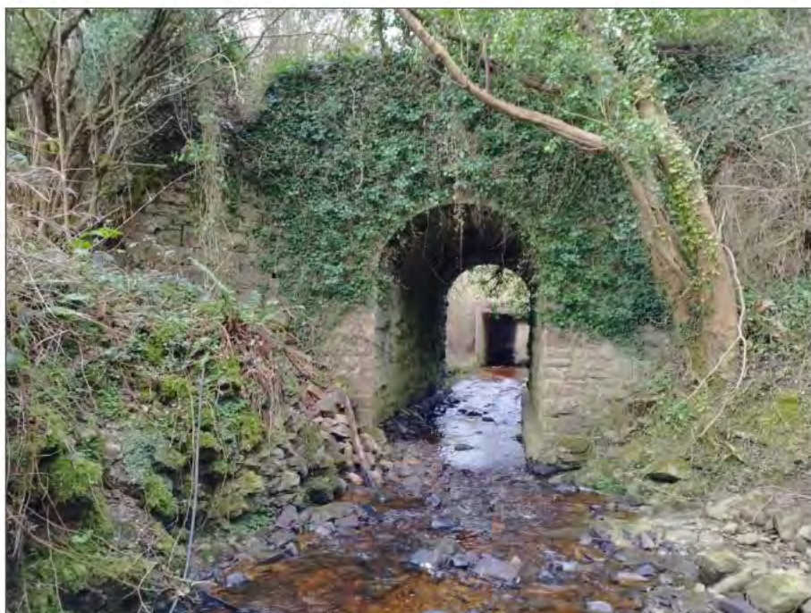
Plate 4-5 Looking downstream from above the masonry bridge.
