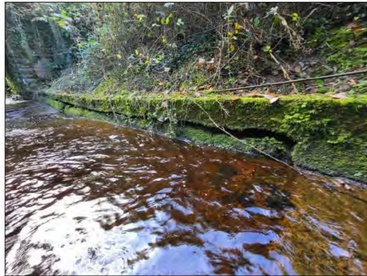
7. EXISTING UPSTREAM TRAINING WALL
