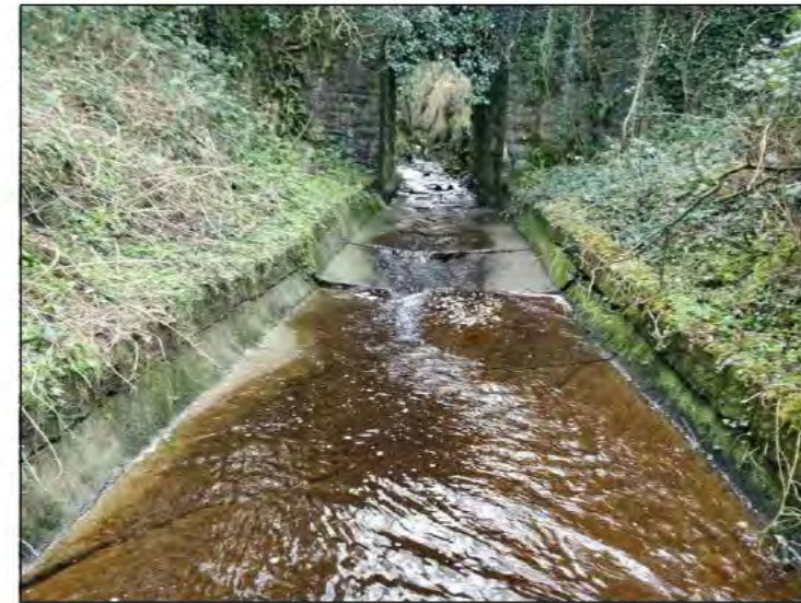
6. UPSTREAM APRON FACING SOUTH
