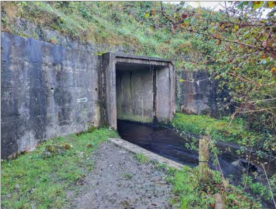
Plate 1-2 Culvert downstream elevation.
