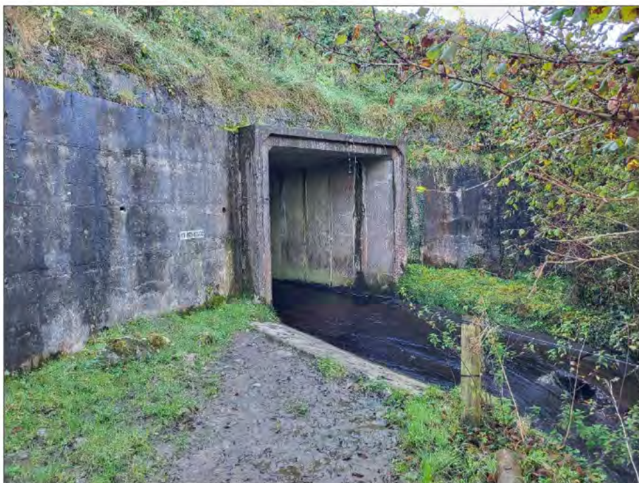
Plate 4-2 Knockbrack Culvert downstream elevation.
