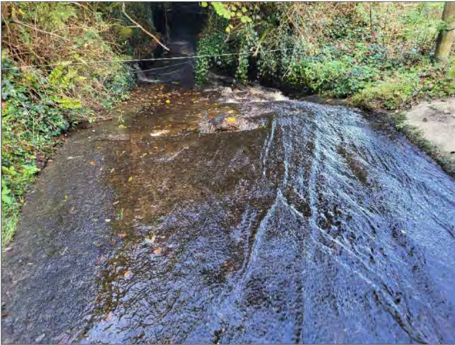
Plate 1-3 Apron downstream of culvert.
