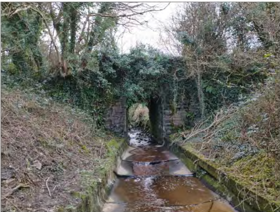
Plate 4-4 Looking upstream from the culvert.
