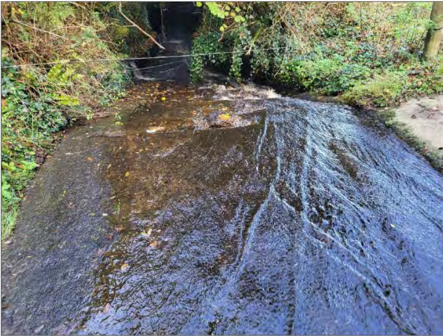
Plate 4-3 Looking downstream from the culvert.
