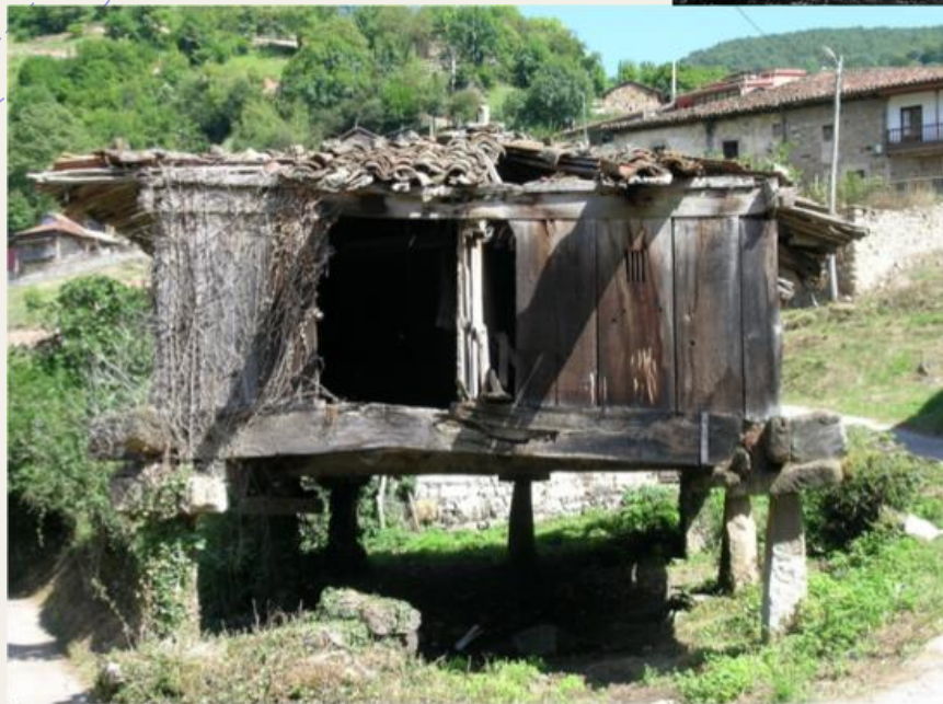
Grain storage structure ( horreo ) in Asturias, Northern Spain (image by Meriel McClatchie)
