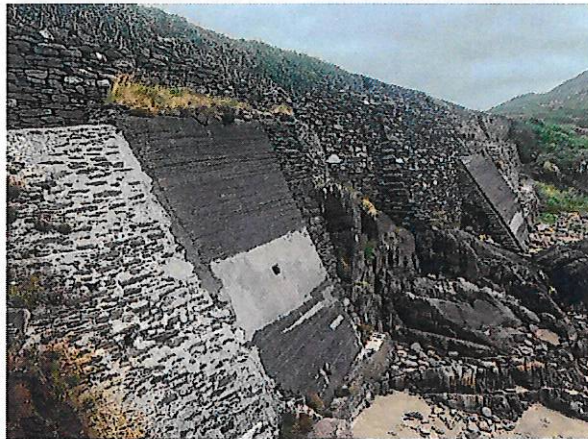
Plate 3. Adjoining areas of rock / retaining wall.
