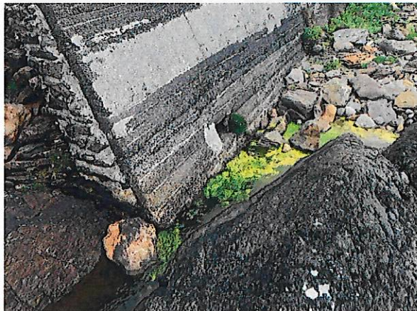
Plate 4. Adjoining areas of rock / retaining wall.
