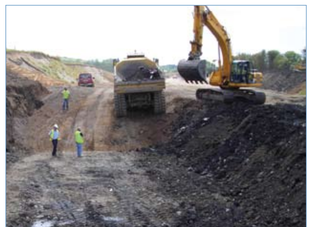
Excavation of Non-Hazardous Waste and Clay (Photograph courtesy of Roadbridge Ltd)
