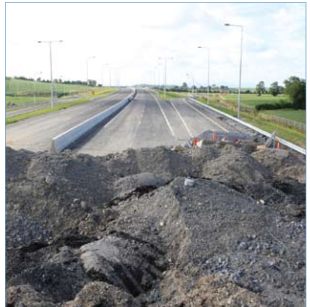
Temporary Storage of Waste Material (Photograph courtesy of Roadbridge Ltd)
