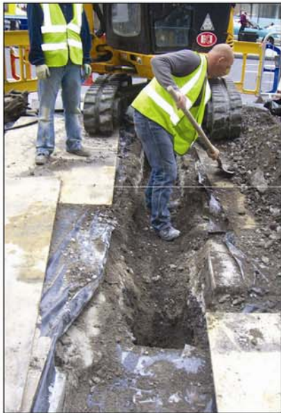
Plate 3 - Mid-excavation of ST719, O'Connell St., west-facing.
