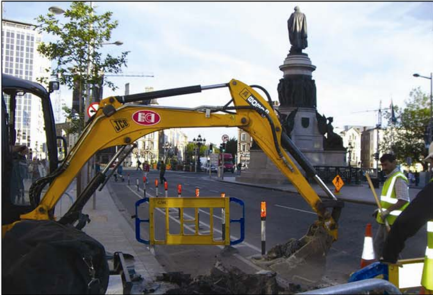
Plate 1 - Mid-excavation of ST715, O'Connell St., south-facing.
