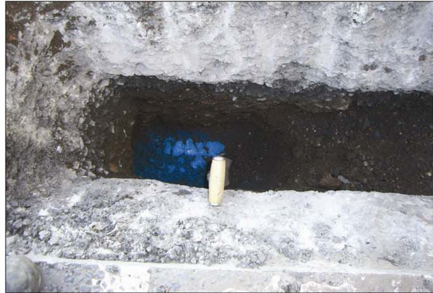
Plate 2 - Mid-excavation of ST715, O'Connell St., south-facing.
