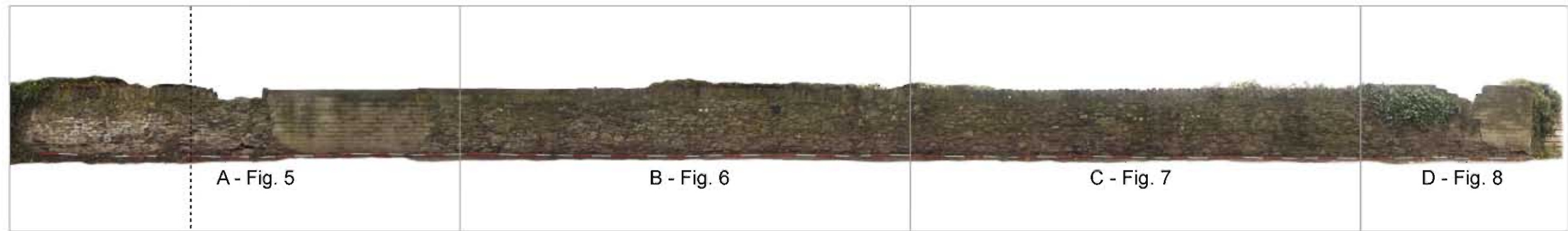
Northeast facing elevation
