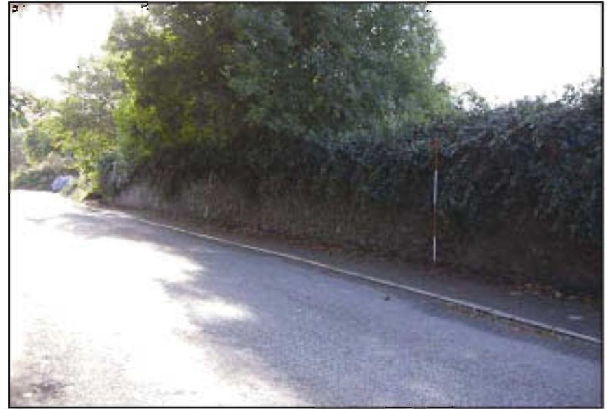
Plate 6 - General view looking southwest along Ennis Lane to townland boundary between Lissenhall Little and Balheary Demesne (HC#414).
