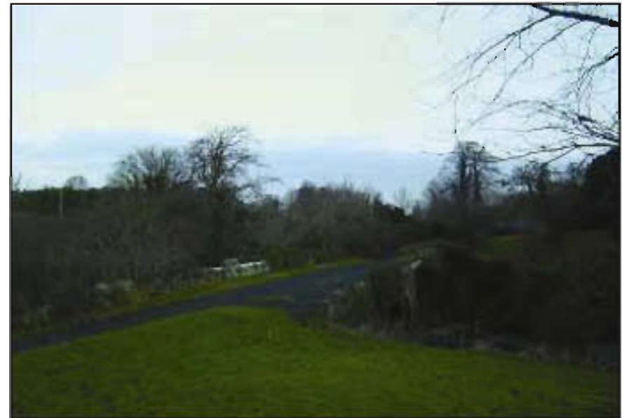
Plate 8 - Photograph of Lissenhall Bridge (HC#11), facing northwest .
