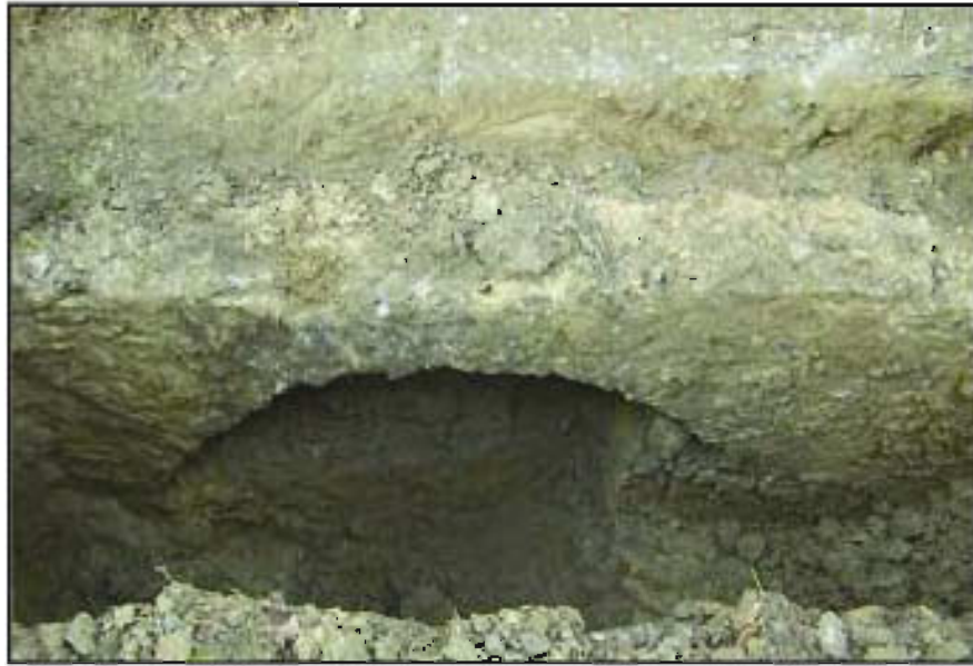
Plate 14 - Photograph of arch/culvert (016) within Test Trench 2, Sub-area 35, facing west.
