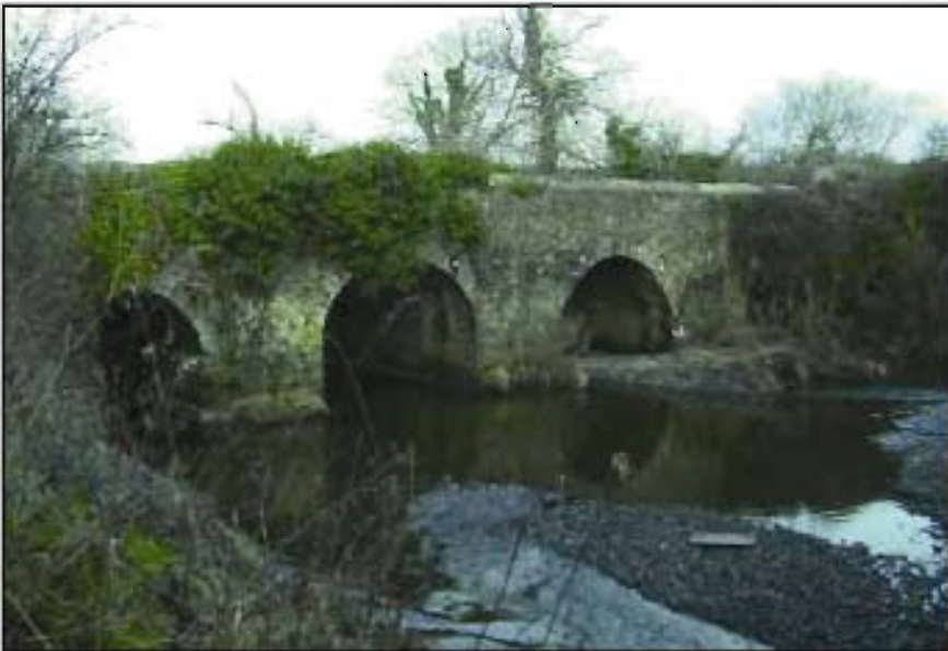
Plate 7 - Photograph of Lissenhall Bridge (HC#11), facing northwest.
