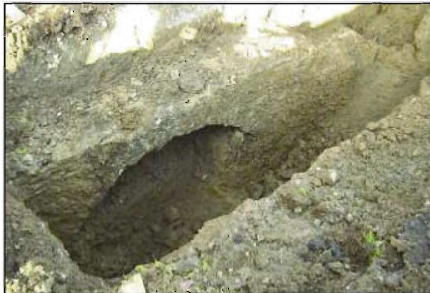
Plate 15 - Photograph of arch/culvert (016) within Test Trench 2, Sub-area 35, facing northwest
