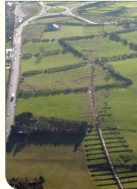
Aerial view of test trenching carried out on the scheme. (Photo Markus Casey)
