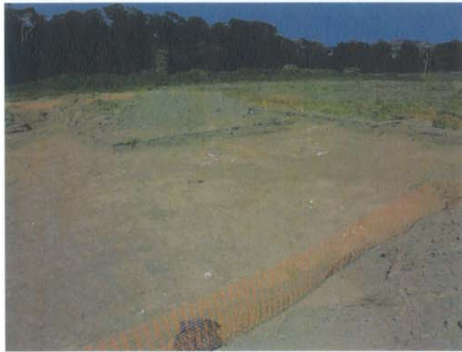
Plate: 5 06E 214, Brenanstown, Site 3A, General site shot, Facing North East
