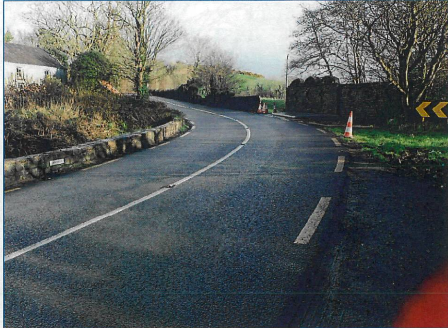
Plate 1. New Court Bridge & N71, facing east [Source: Atkins R.E.].
