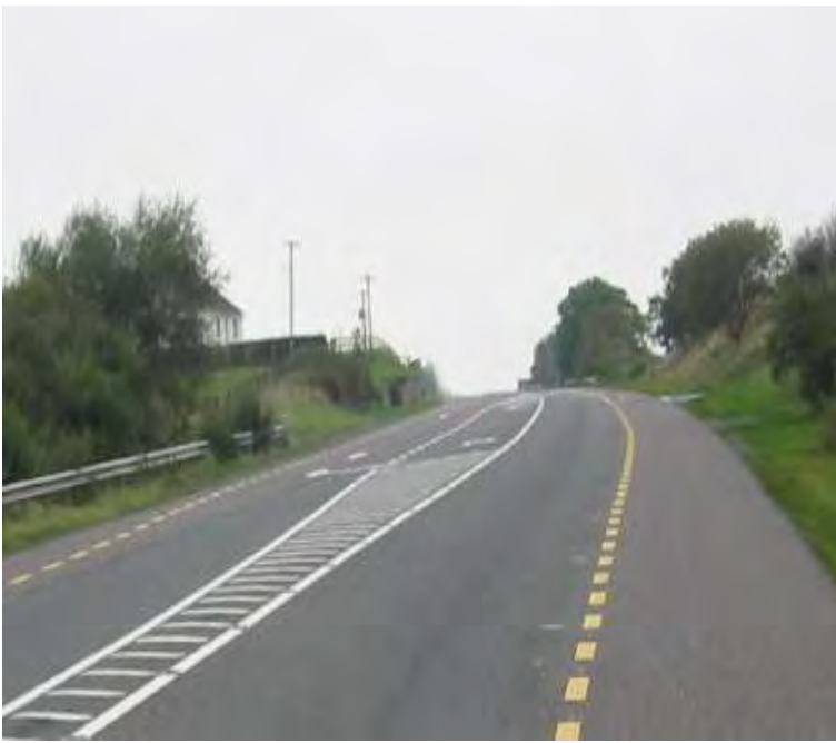
After road safety remedial measure implemented
