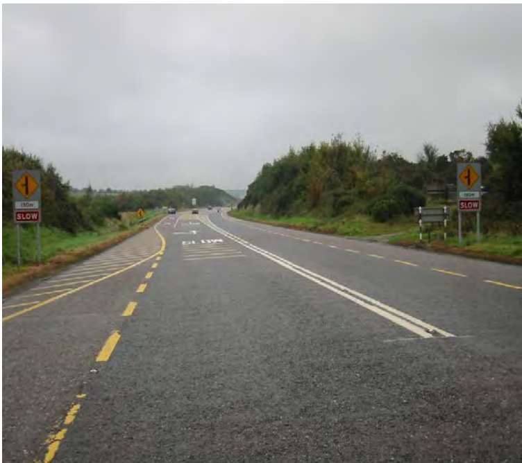
After road safety remedial measure implemented
