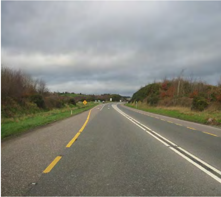
Before road safety remedial measure implemented
