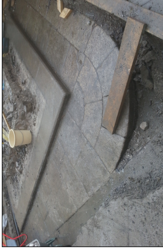
Plate 7: Westmoreland St.; Thomas Moore statue; view of old street paving following removal of statue.
