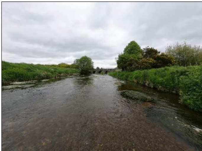
Plate 2 River Slaney looking upstream to Rathvilly Bridge from downstream survey extent, June 2019.
