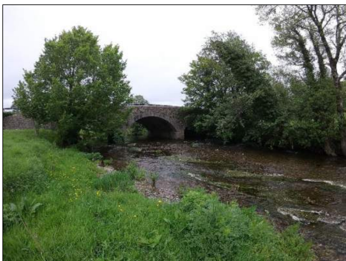
Plate 5 River Slaney at Eldon Bridge, June 2019. Freshwater Pearl Mussel (FPM) habitat was also considered suboptimal at this survey stretch due to substrates present. No live FPMs or dead shells were recorded.
