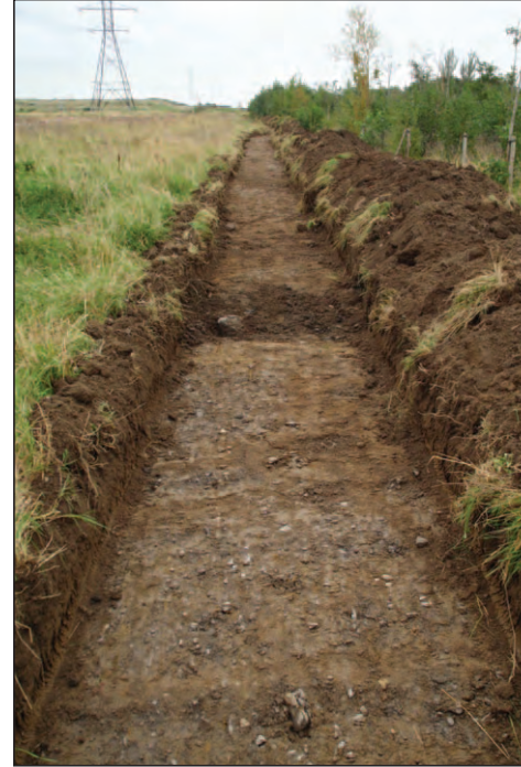
Plate 2 - Testing area 2, trench 2, water mains trench, (003), facing northeast.
