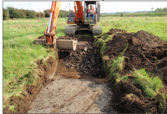
Plate 4 - Testing area 2, trench 5, (013), modern stone filled drain, facing east
