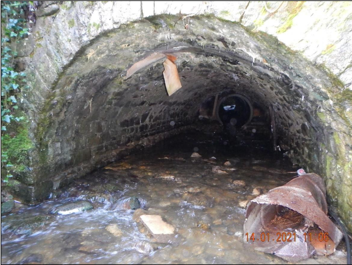
Plate 2. Masonry arch barrel and concrete pipe culvert.
