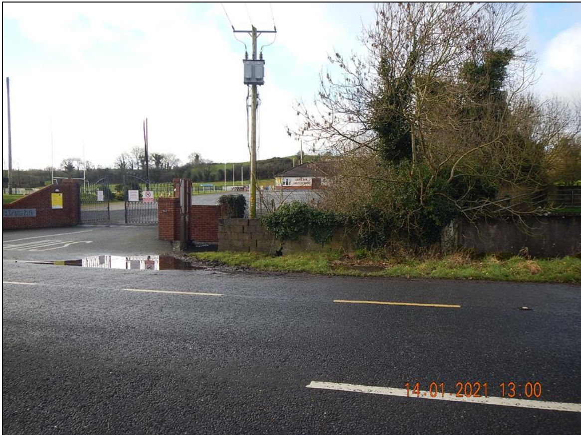
Plate 4. Bridge deck and western blockwork parapet.
