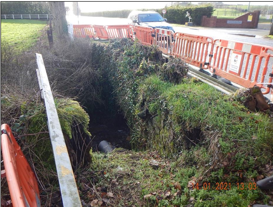
Plate 3. Eastern side of structure.
