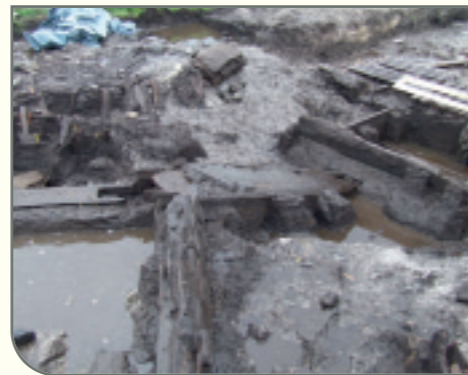
View of millpond, flume and undercroft of Kilbegly Mill. (Photo: Studio Lab)
