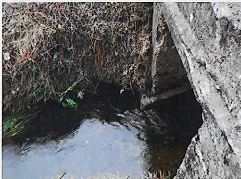
Plate 3. Upstream of Coolloughra Bridge. [Source: Atkins R.E.; 08/01/2019]
