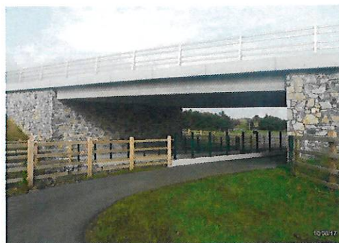
Plate 4. Parapet beam showing no outfall.
