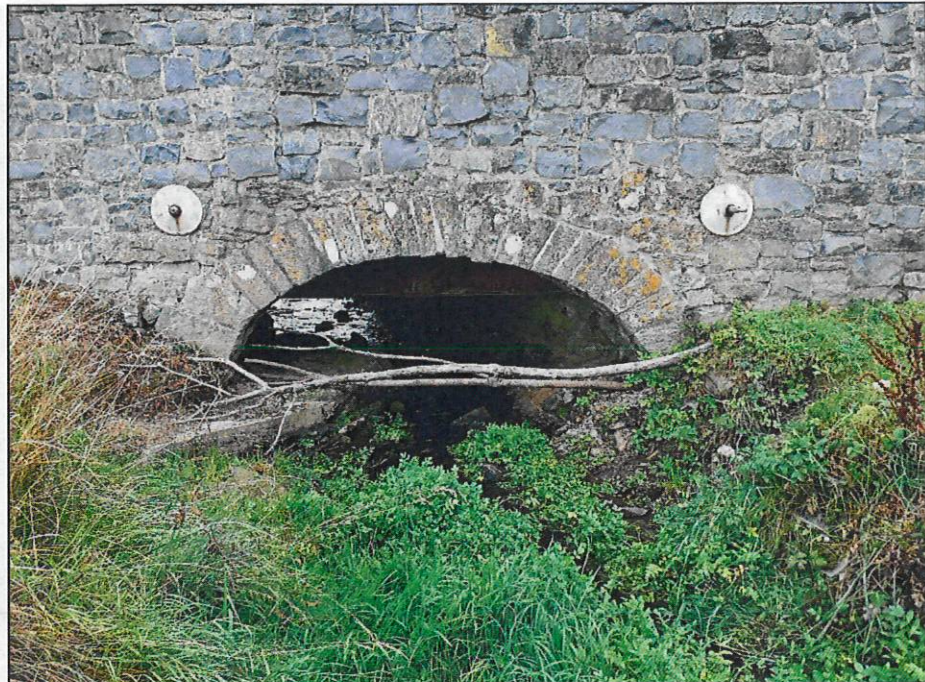
Plate 1. Upstream side of bridge, facing downstream.
