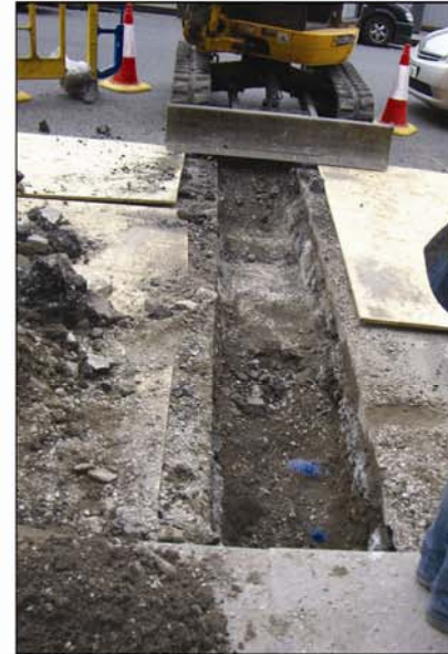
Plate 2 - Mid-excavation of carriageway ST729, Stephens Green north, southwest-facing.
