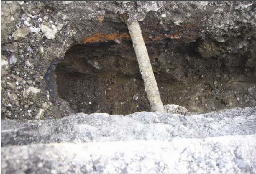
Plate 1 - Mid-excavation of ST728 showing utilities, Stephens Green north, northeast-facing.
